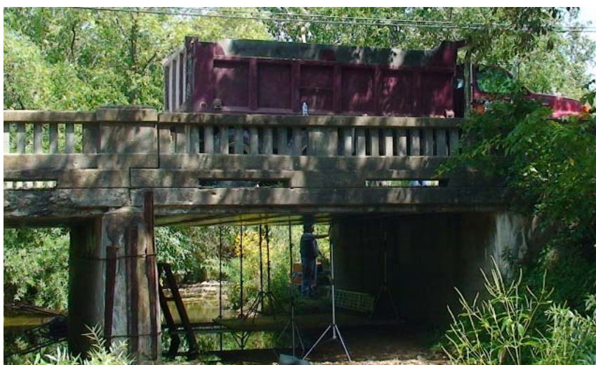
Figure 3-4 Load Test with a H20 Truck
