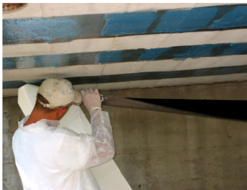
(c) Application of CFRP laminates
