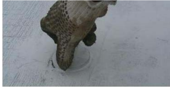
(b) Removing Dummy Casing
