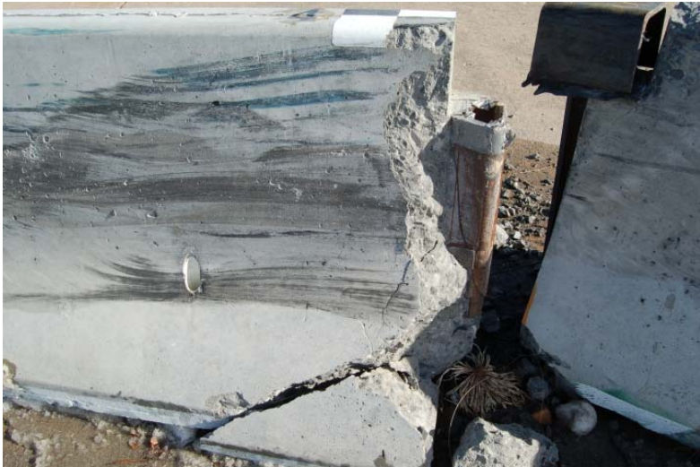
Figure 26. Barrier No. 4 Damage, Test NYTCB-4
