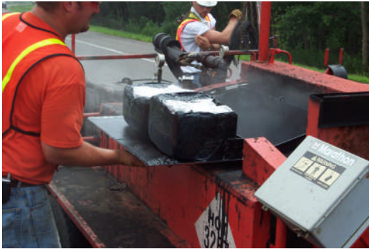
Photo 1: Loading Adhesive into Melting Pot
