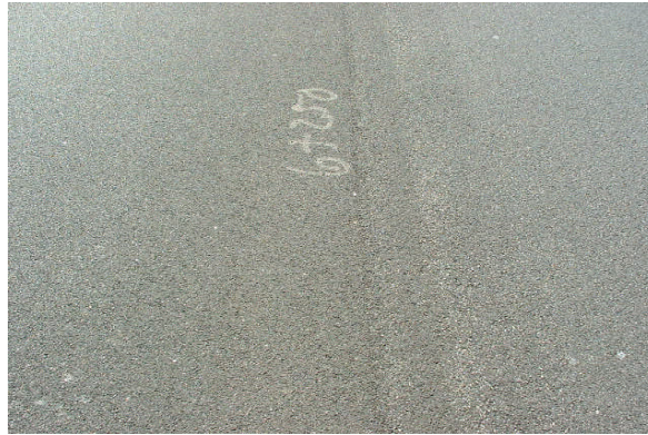
Photo 13: Good Centerline Seam – Route 3
