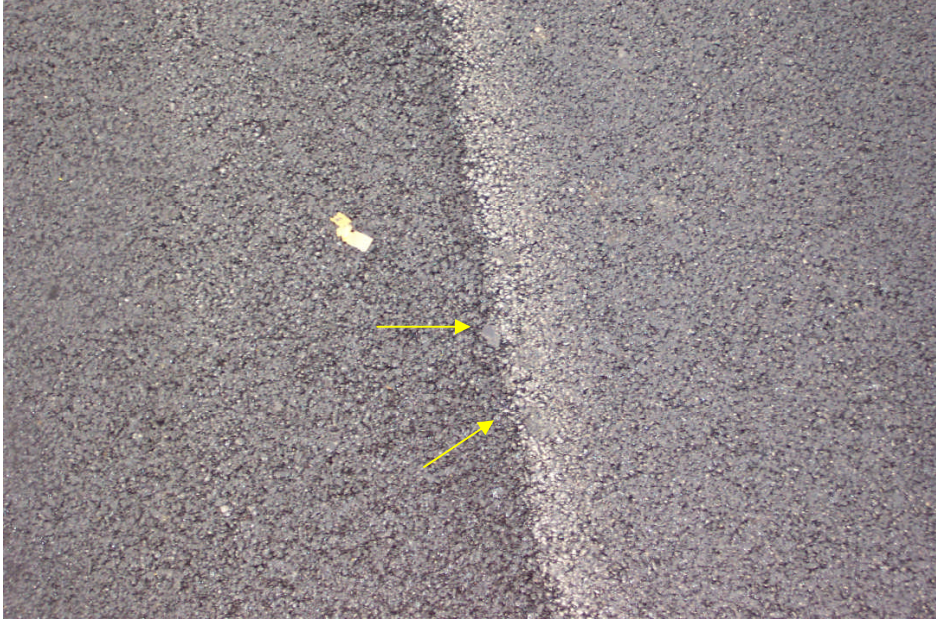
Photo 9: Adhesive Beads @ Surface After Rolling
