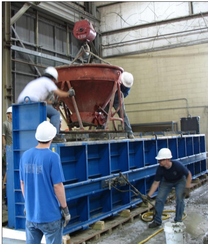
Figure 3-16: Concrete Placement and Form Vibration
