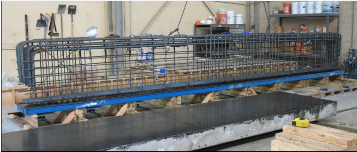
Figure 3-13: Instrumented Reinforcement Cage on Form Soffit
