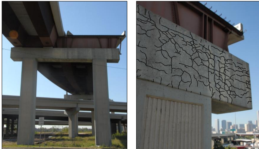
Figure 1-1: US 59 and I-10 Interchange - Houston, Texas
