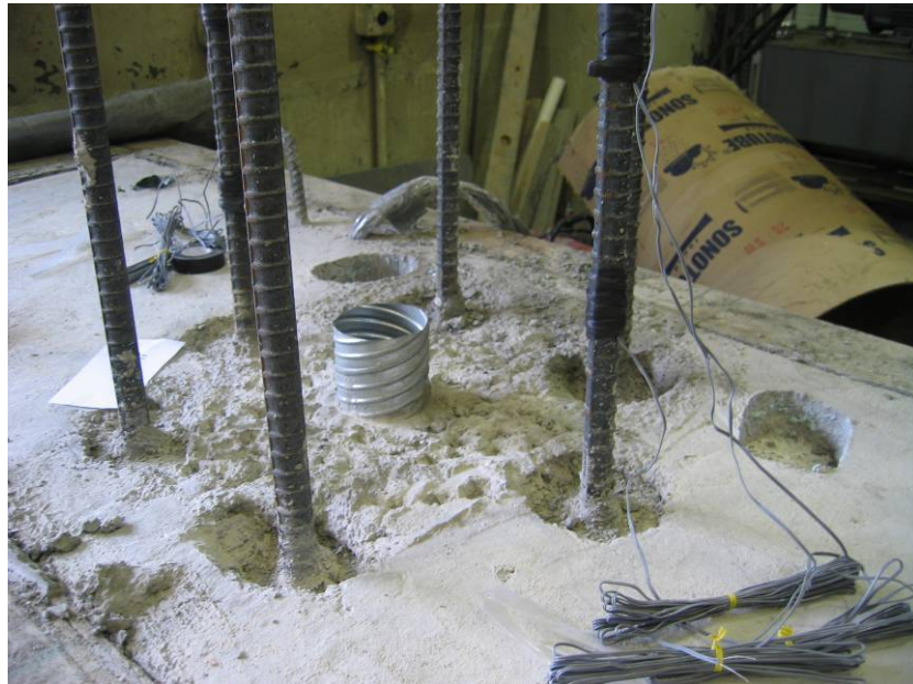
Figure 3-2. Specimen LB7-PT cap-beam after casting.
