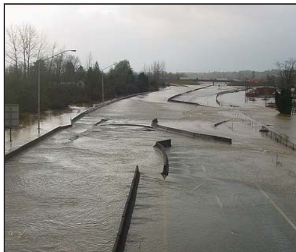
I-5 damage resulting from the severe flooding
