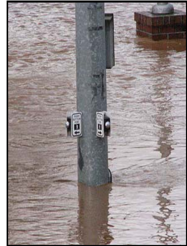
A pedestrian signal nearly submerged by the Lewis County floodwaters
