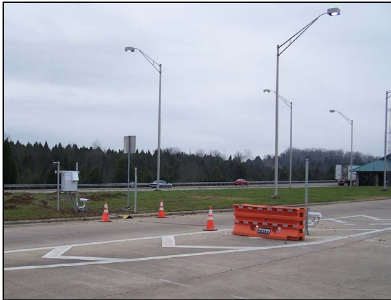
Figure 3. Photo. Location of SIRIS system.
