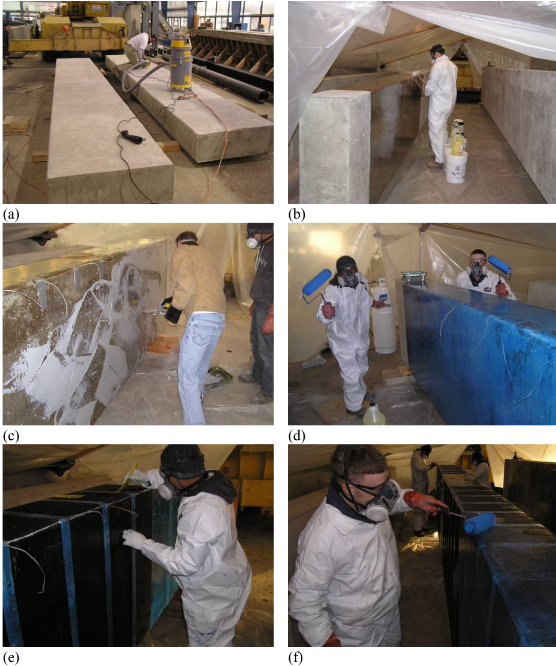
Figure B-4.3: CFRP application process
