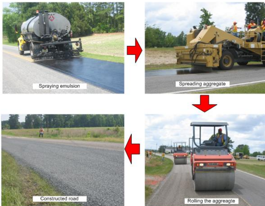
Figure 2-2 Chip seal construction procedure
