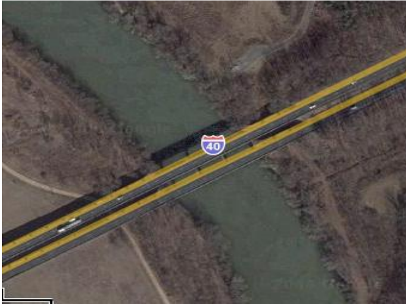
Figure 18 Yadkin River Bridge
