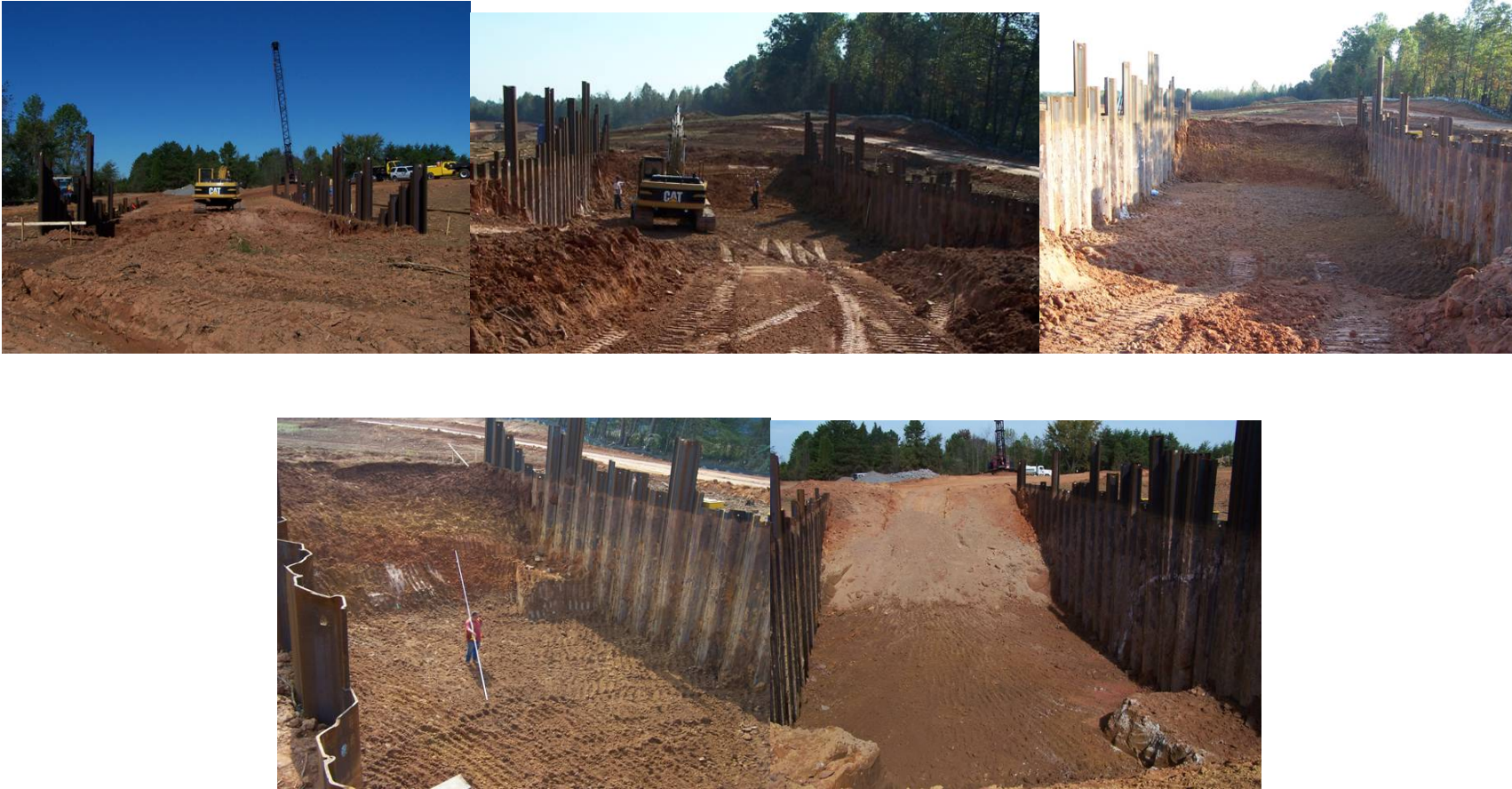
Figure 5.10 – Photographs of excavation in Statesville
