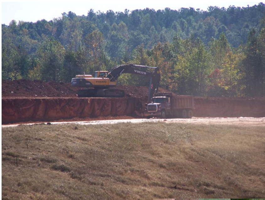
Figure 6.4 - Vertical excavation of soil onsite
