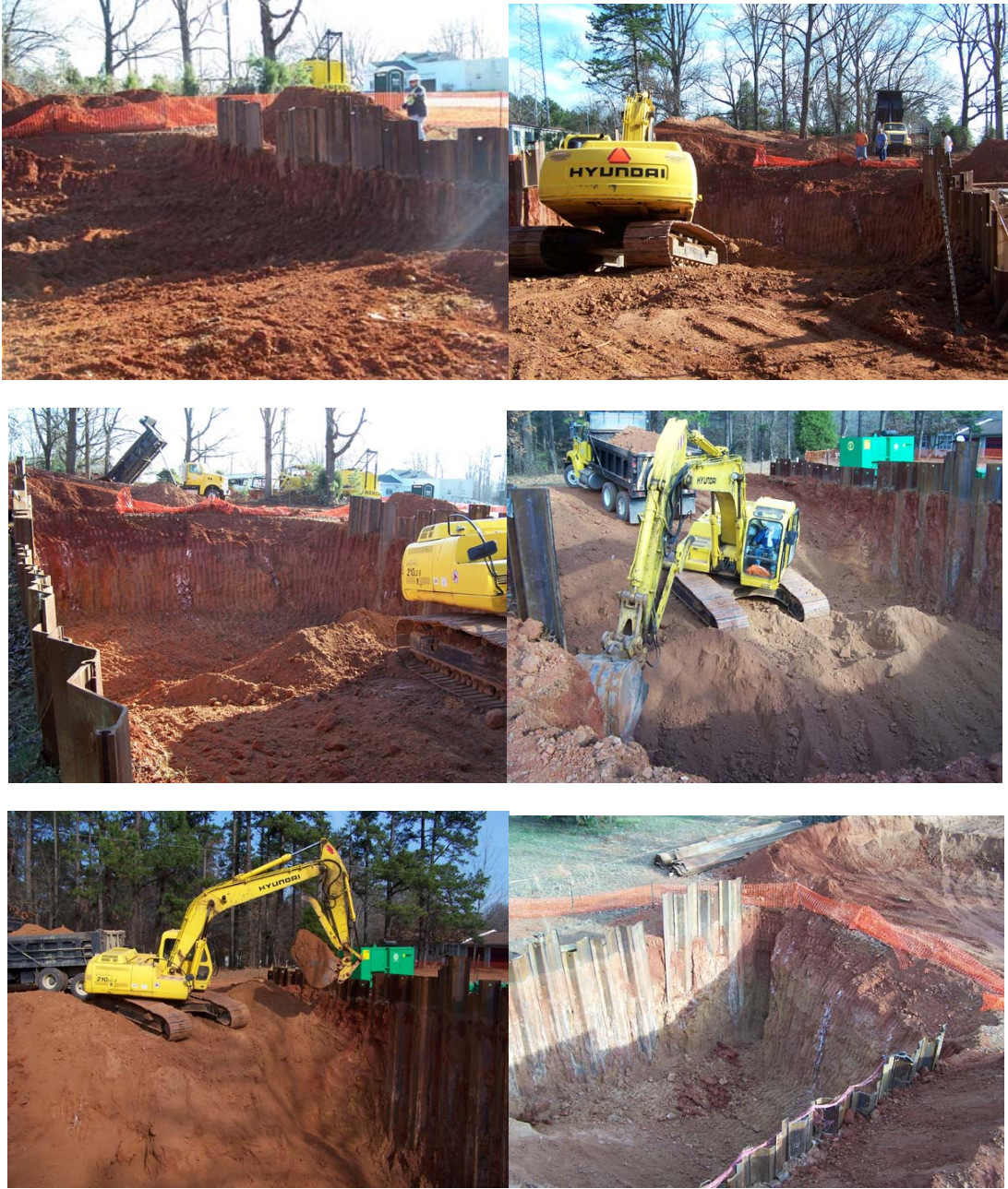
Figure 5.17 – Photographs of excavation in Monroe
