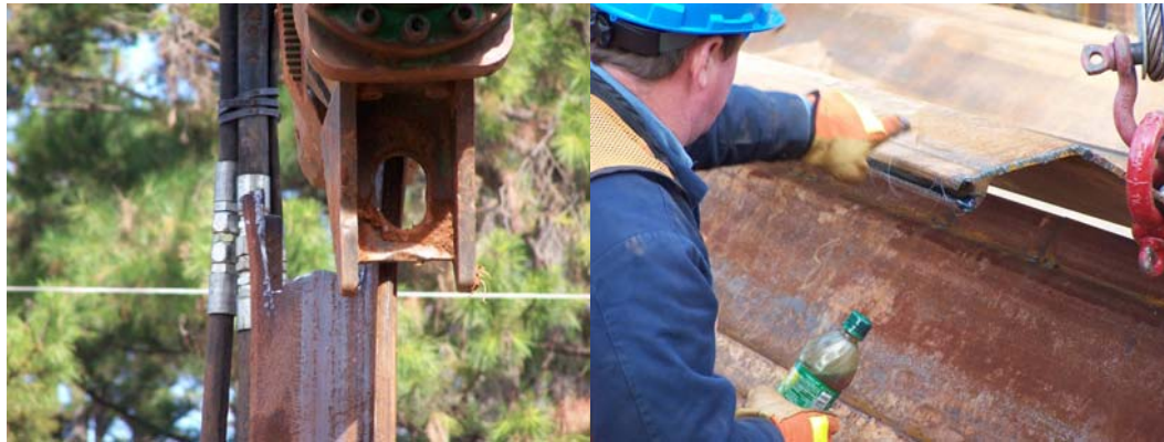
Figure 5.13 – Photographs from wall installation in Monroe
