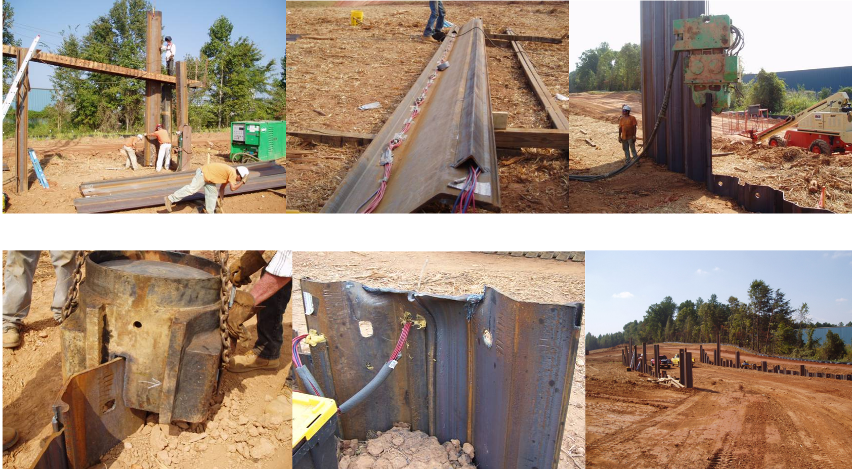
Figure 5.7 – Photographs from wall installation in Statesville
