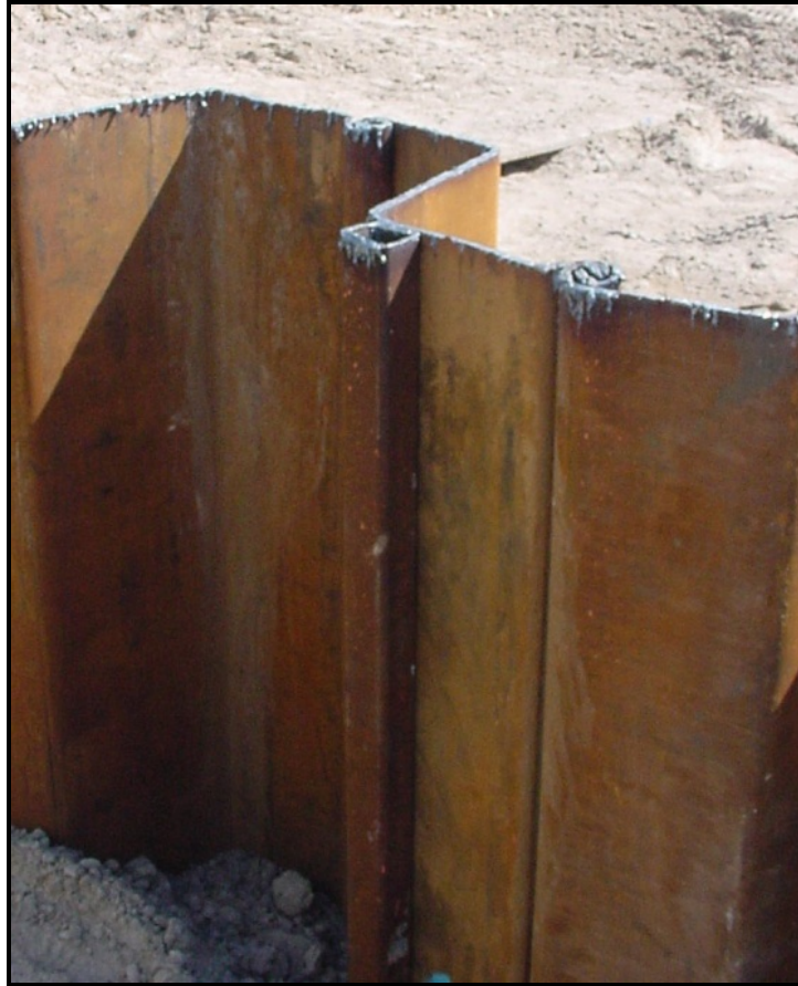
Figure 5.3 - Steel tube welded to a sheet pile as an inclinometer casing
