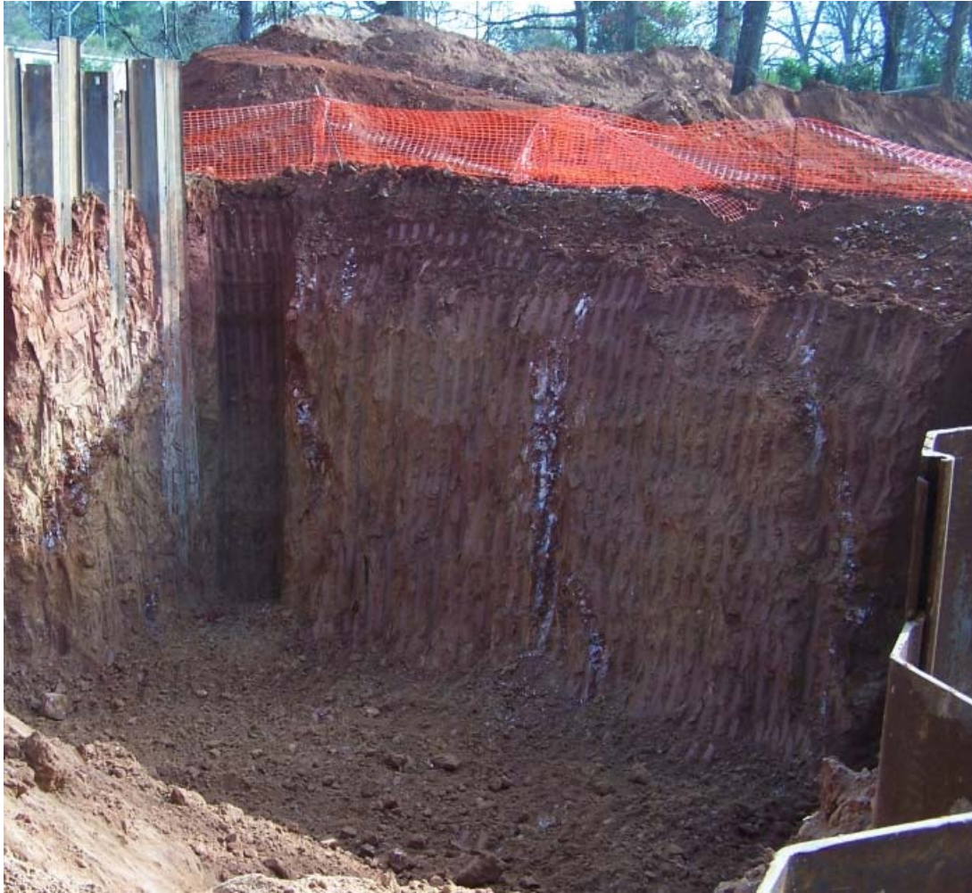
Figure 6.8 - Unsupported soil mass (20ft excavation)
