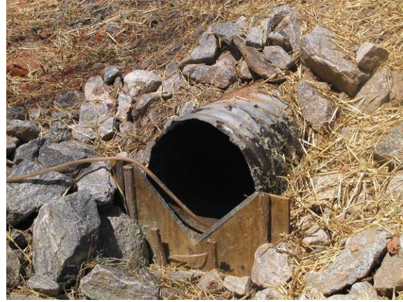
Figure 13. Weir at Fleming Chapel.
