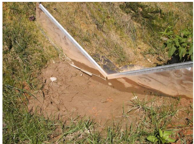
Figure 11. Weir at Steeltown Rd.
