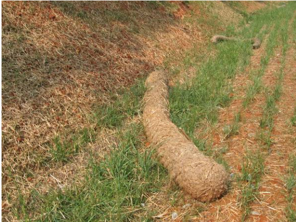
Figures 3 and 4. Examples of coir logs.
