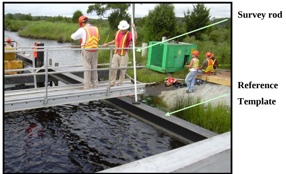
Figure 5-17 Beginning to perform pre-jet survey.
