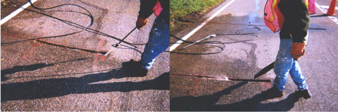
Figure 59 Photograph showing the power washing and blowing of the groove to remove debris and water.
