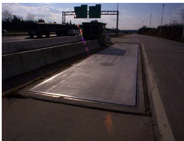
Figure 49 Route 287 weigh station static scale.
