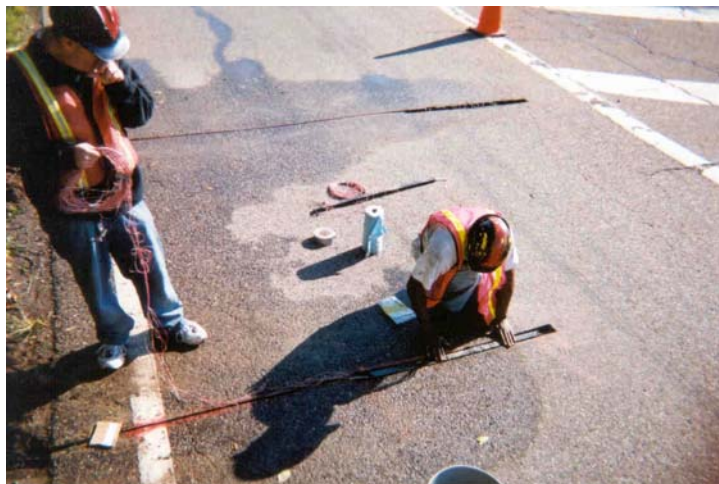
Figure 61 Photograph of ceramic-polymer composite sensor assembly being placed in groove at the Route 287 weigh station.
