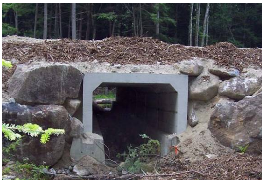
(a) flat-top ( www.americanconcrete.com )
