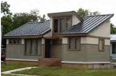
Solar Homes under construction
