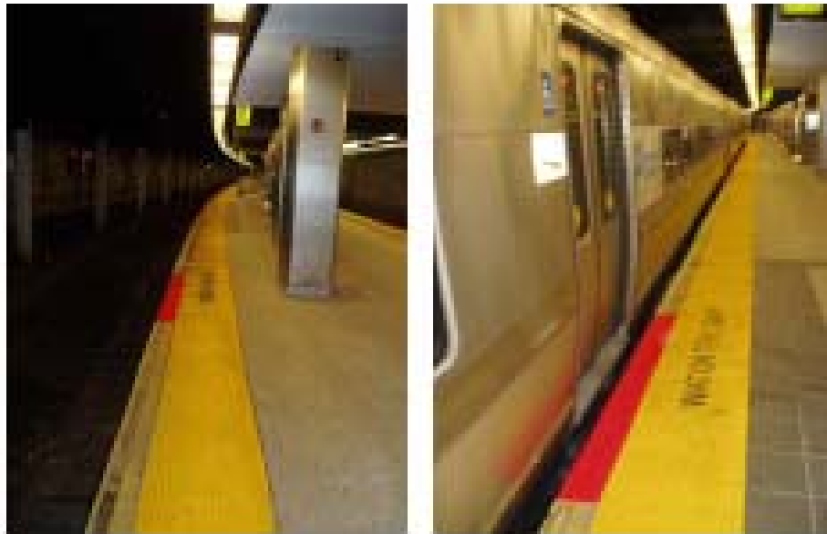
Figure 2. LIRR Flatbush Ave. Station with Red Lines Underscoring Wider Gap
