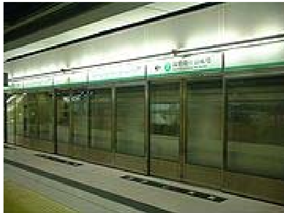
Figure 7. Platform Screen Doors at Hong Kong's Tiu Keng Leng Station
