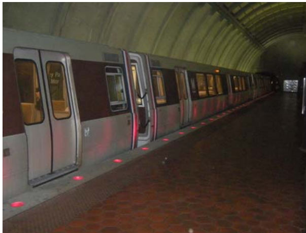
Figure 35. Washington D.C. Platform Edge Lights
