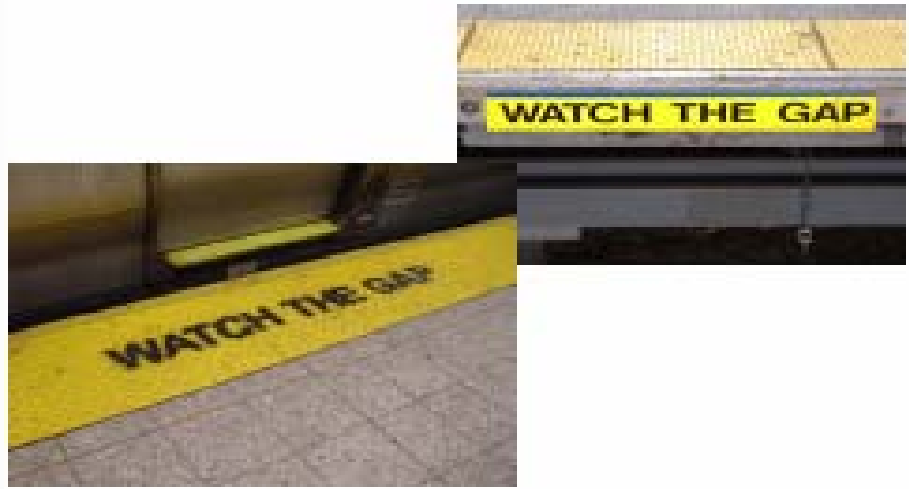
Figure 3. LIRR stencils “Watch The Gap” to Yellow Lines
