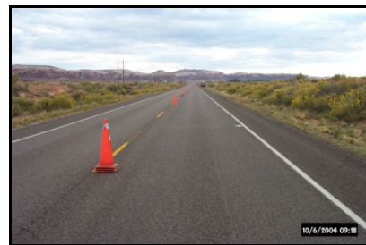
Newly constructed HMA (initial IRI)
