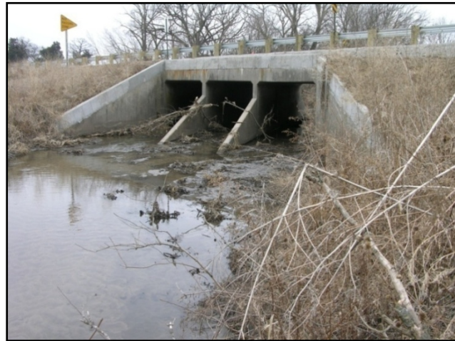
Figure 2-1-1 Typical Iowa culvert (near Solon, Iowa)
