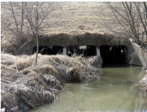
The effect of the long term sedimentation is obvious (with trees already growing on the new deposits)
