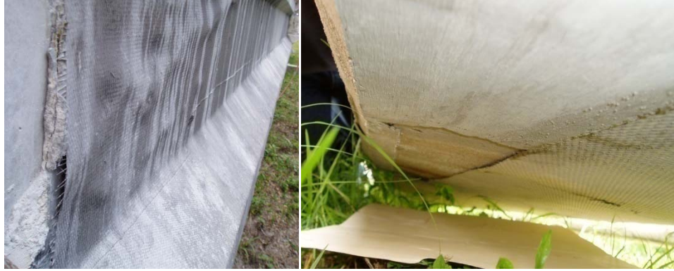
Figure 1: Beams Removed from I-95 Bridge
