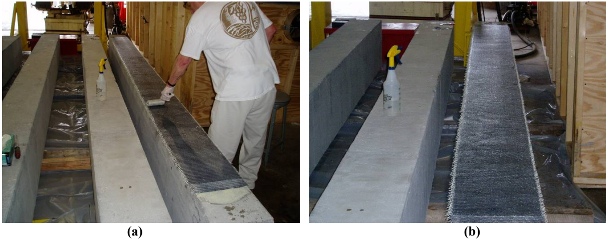
Figure 12: Installation of PU-System
