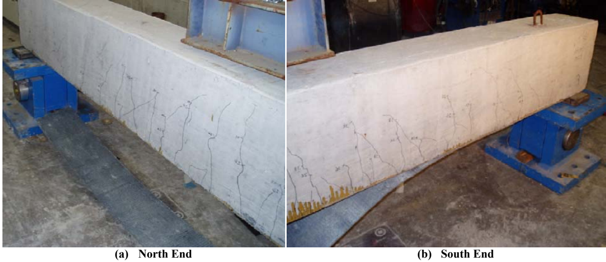
Figure 70: PU-T at Failure
