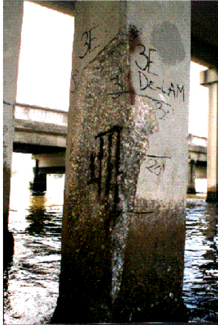
Figure 1: Photograph of a coastal bridge spalled piling.
