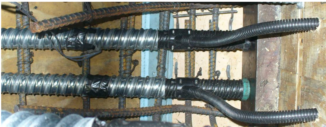
Figure 94 – Galvanized steel duct, HDPE duct at anchor plate, and HDPE grout tubes.
