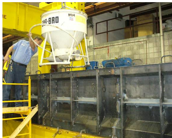
Figure 91 – Welded steel girder formwork
