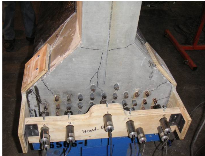
Figure 25 – Cracking at support and strand instrumentation.
