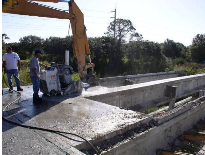
Figure 32 – Deck cutting operation in preparation for girder removal.
