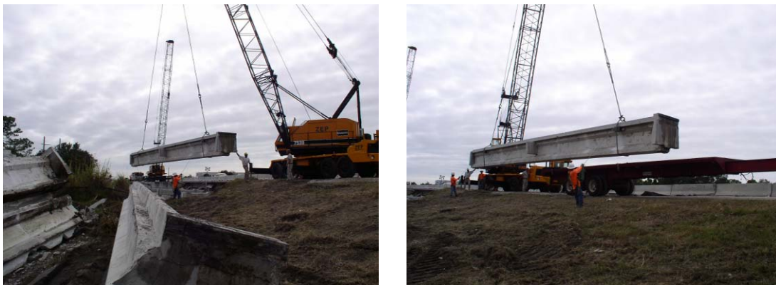
Figure 33 – Removal of Type III girders.
