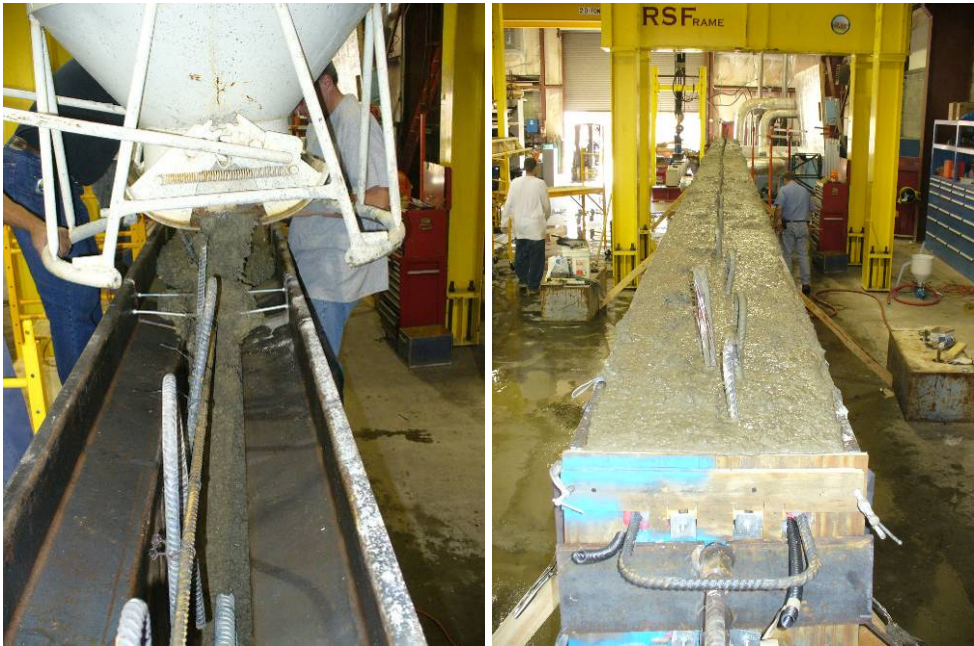
Figure 98 – Girder concrete placement.
