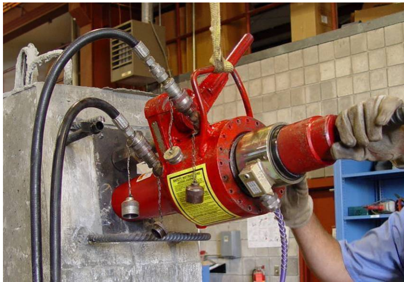
Figure 102 – Hydraulic jack used to stress PT bars.
