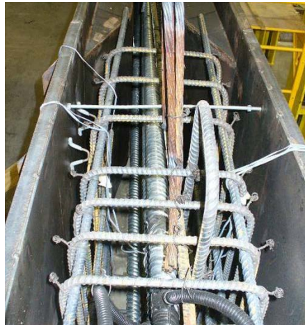
Figure 93 – End block reinforcement resting against a chair.
