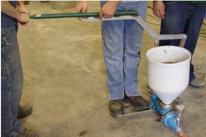
Figure 99 – Grout injection using hand pump.
