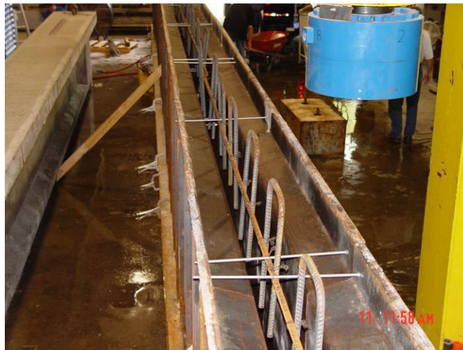
Figure 97 – U-bar positioning.
