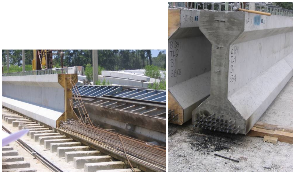
Figure 7 – Prestress transfer and girder ready for shipping.
