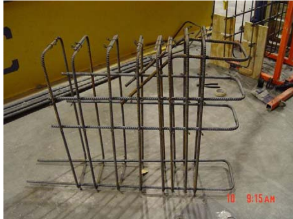
Figure 92 – End block reinforcement cage.
