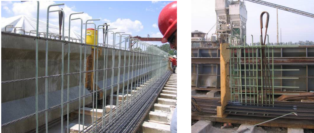
Figure 6 – Reinforcement and prestressing placement
