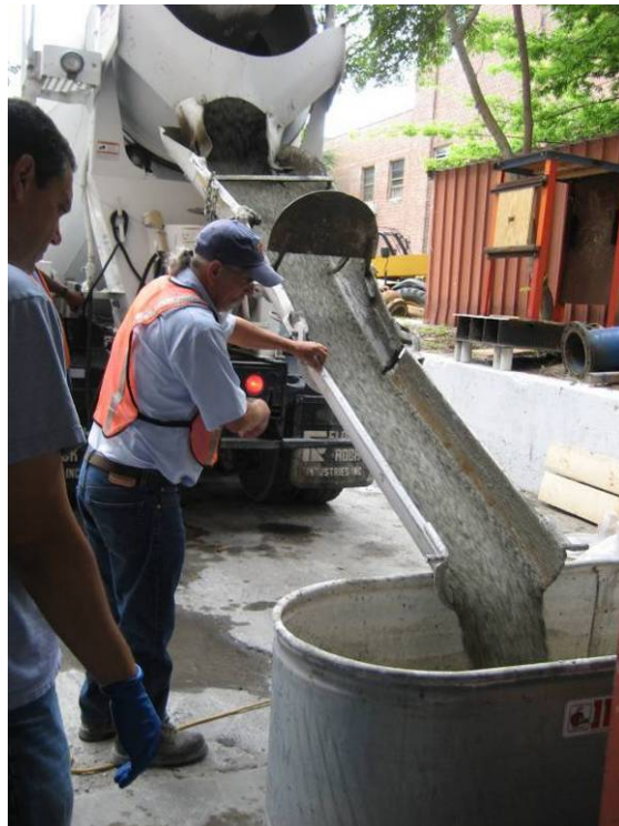
Figure 14. Ready-mixed concrete being discharged into the container for transporting.
