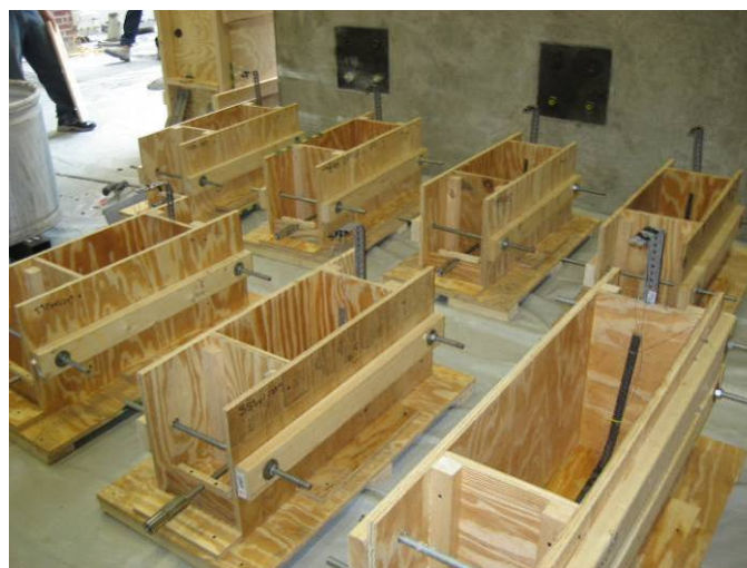
Figure 13. Photo of formwork ready for concrete placement.
