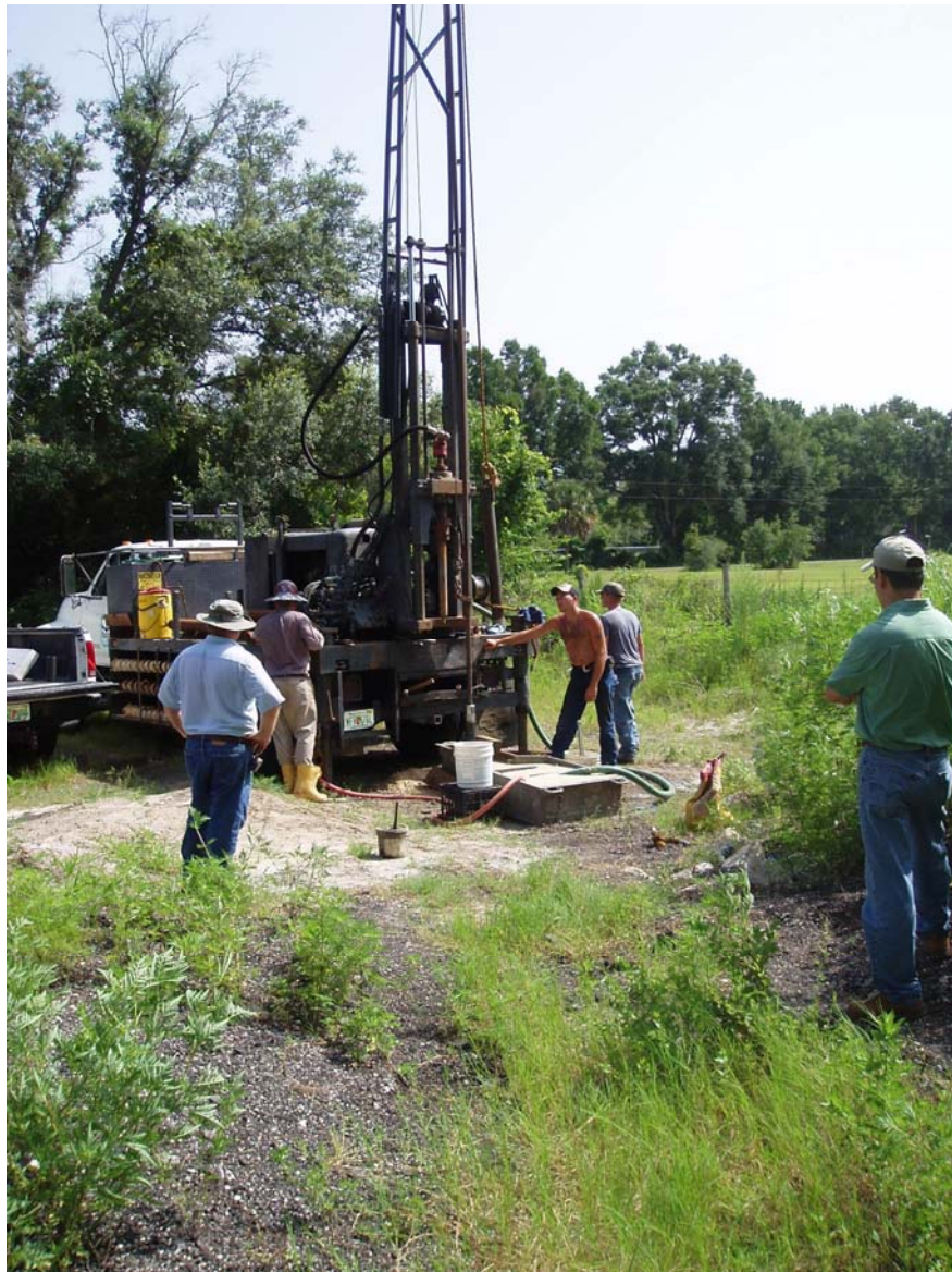
Figure 6-14. Field Coring at the Kanapaha Site.
