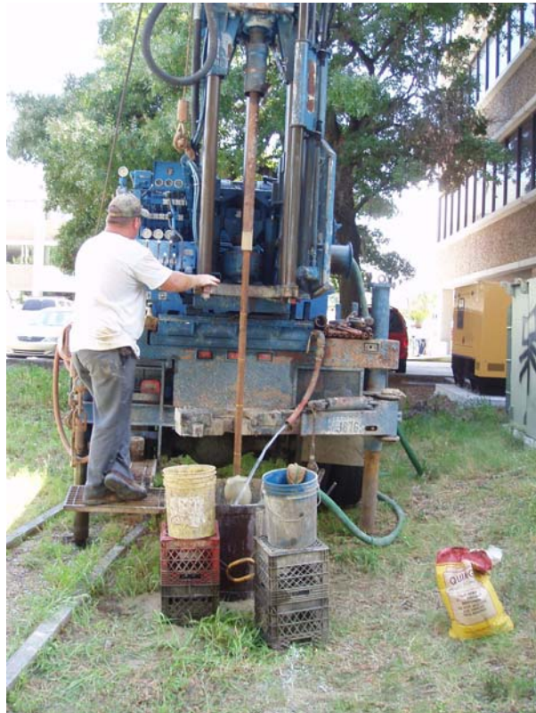
Figure 6-3. Coring at the Fuller Warren Bridge Site.
