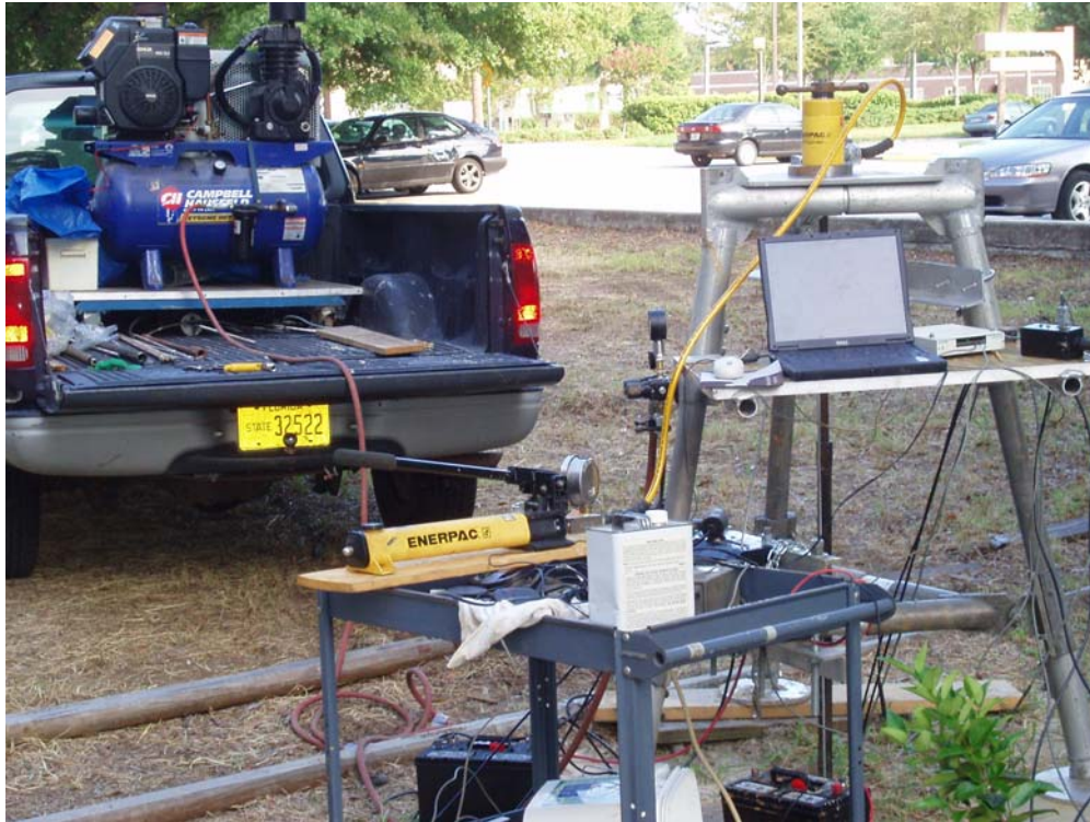
Figure A-18. Field Setup of Compressor, Jack and Data Collection System.
