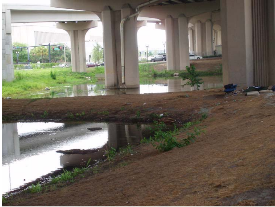
Figure 6-2. Piers at the Fuller Warren Bridge Site.
