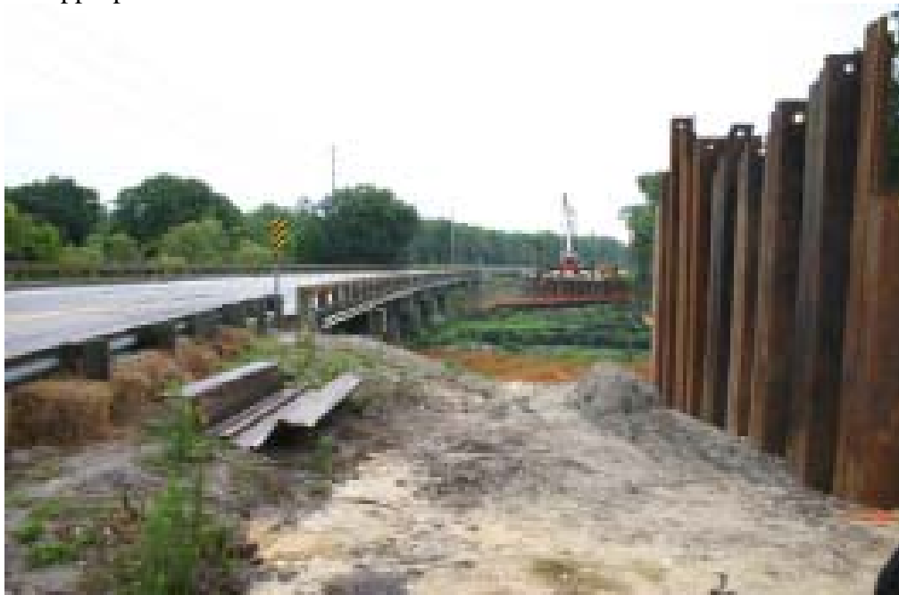
Figure 1.1 Cantilevered sheet pile wall adjacent State Road 39, Hillsborough County.
