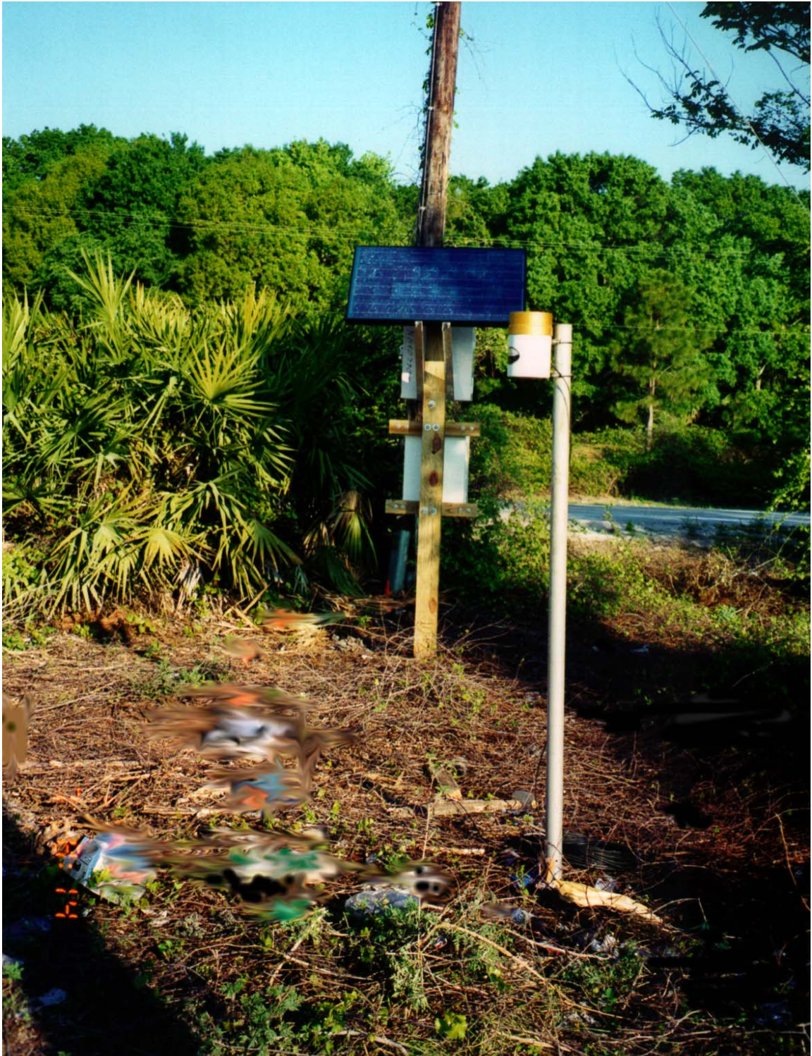
Figure B.4 Rain Gauge Installation in Field Test Sites
