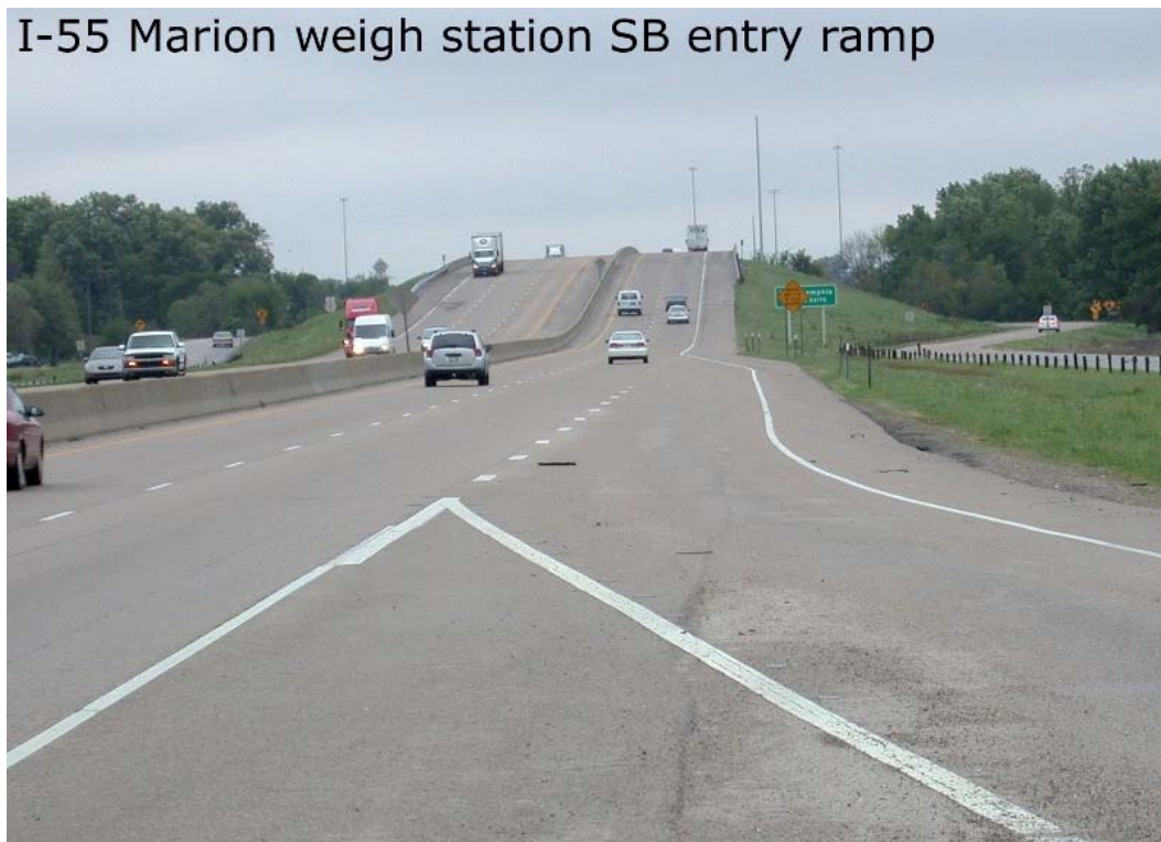
Figure 3-10: Marion Weigh Station Freeway Acceleration Lane
