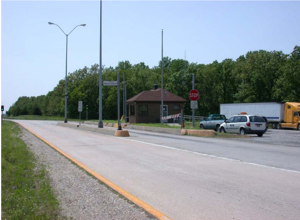
Figure 3-5: Joplin Weigh Station Building and Static Scales
