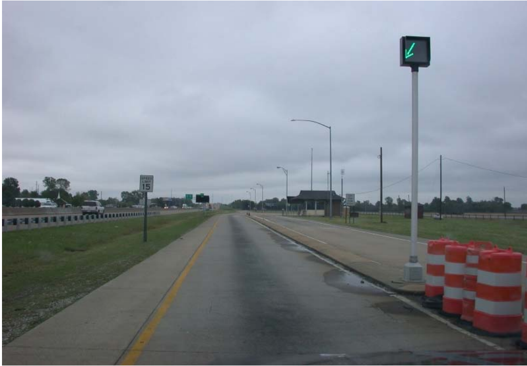
Figure 3-9: Marion Weigh Station Building and Static Scales
