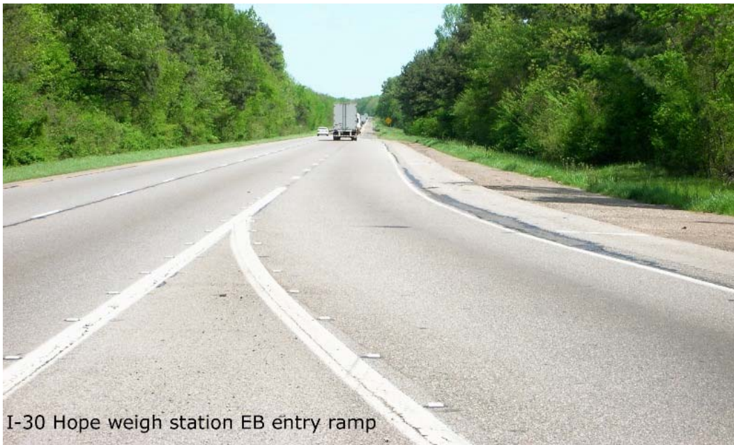
Figure 3-4: Hope Weigh Station Freeway Acceleration Lane
