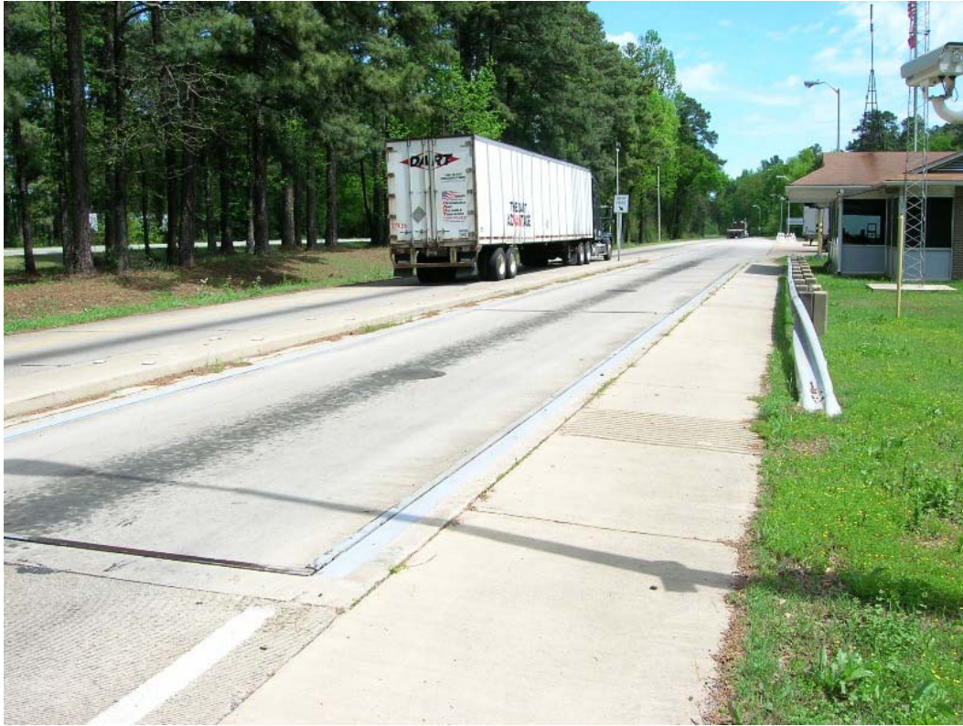
Figure 3-3: Hope Weigh Station Building and Static Scales
