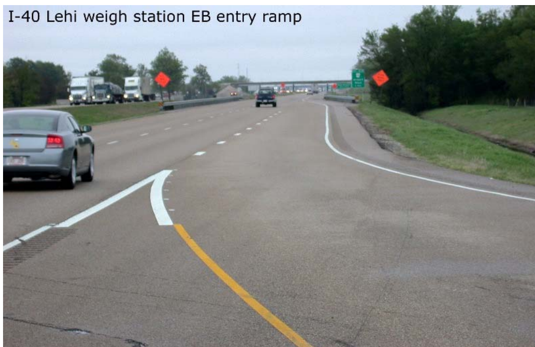
Figure 3-8: Lehi Weigh Station Freeway Acceleration Lane
