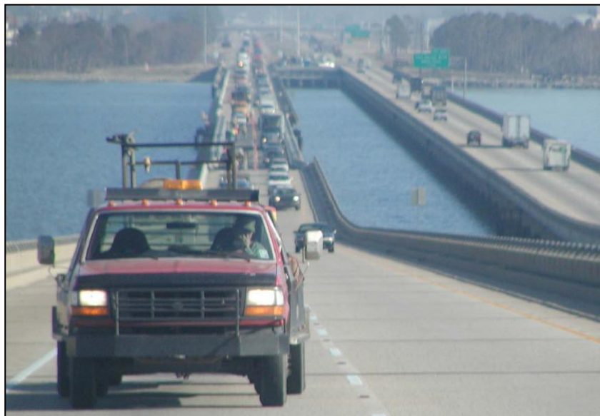
Figure A-39. Project finished and beginning phase III (Courtesy of LADOTD and Paul Fossier)
