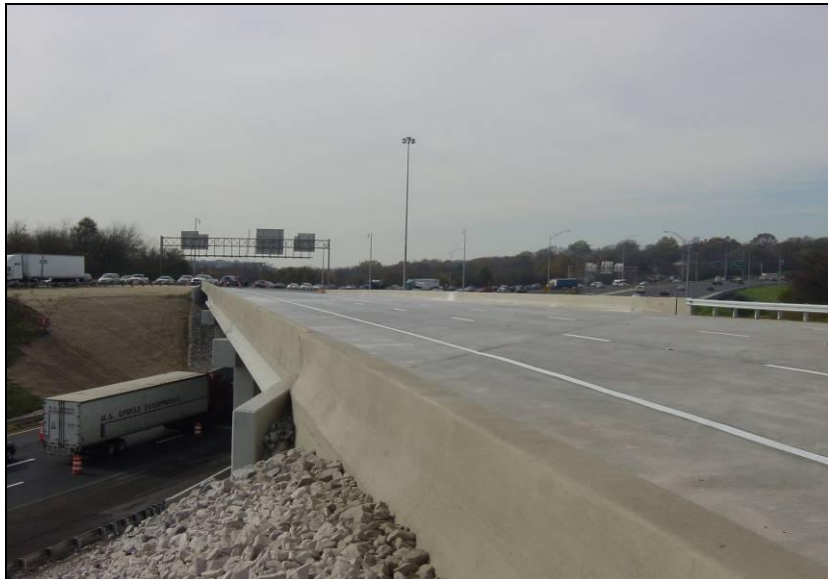
Figure A-12. Fifth week: completed I-59/20 bridge (Courtesy of Brasfield & Gorrie)
