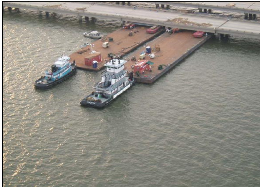
Figure A-35. Lifting spans (Courtesy of LADOTD and Paul Fossier)
