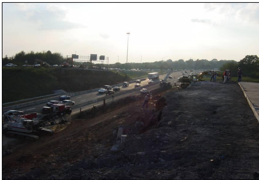
Figure A-7. Clean up of I-20/I-59 bridge (Courtesy of Brasfield & Gorrie)
