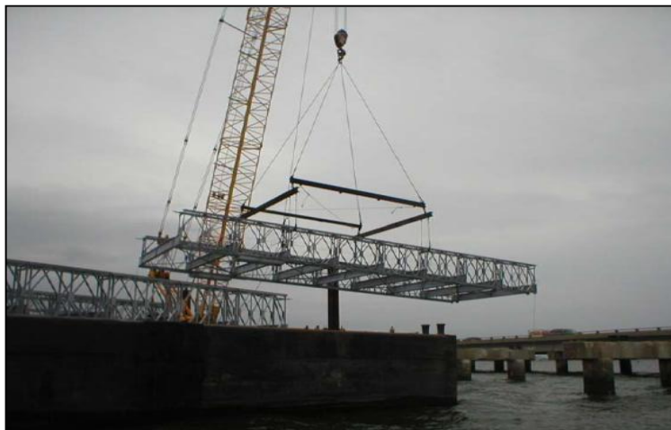
Figure A-37. Acrow 700 series steel panels (Courtesy of LADOTD and Paul Fossier)
