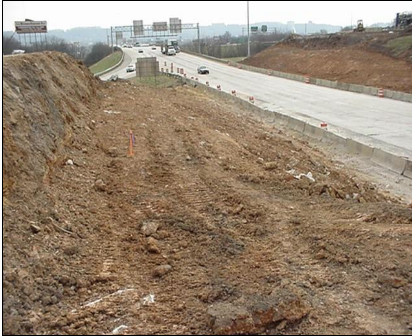
Figure A-1. Beginning the I-65 bridge replacement (Courtesy of Brasfield & Gorrie)
