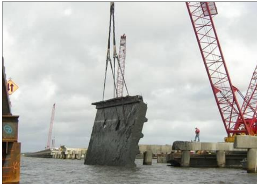
Figure A-26. Spans removed from water (Courtesy of FDOT and William Nickas)
