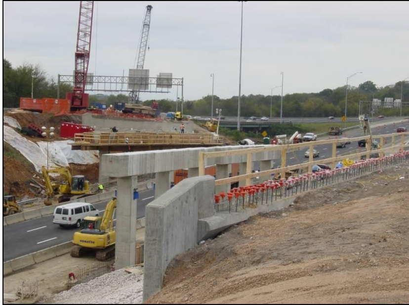
Figure A-9. Second week: concrete caps and columns (Courtesy Brasfield & Gorrie)
