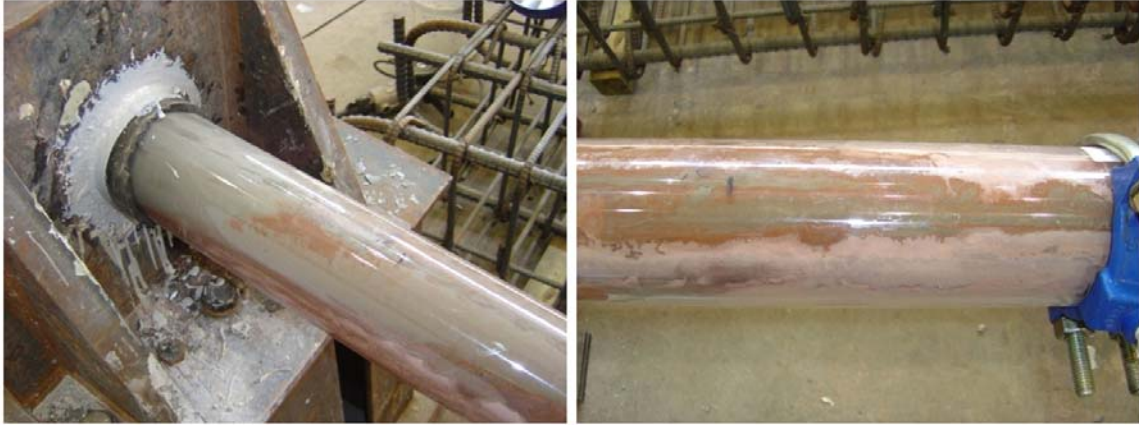
Figure B-43. Repair Grouted Ducts of Specimen PVG-C3-1.
