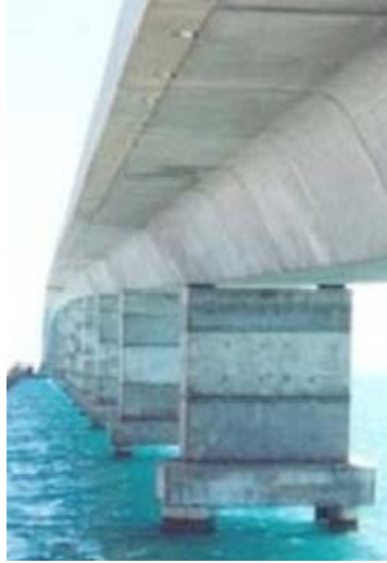
Figure 2-2. Niles Channel Bridge, Florida Keys, Florida (Structurae 2009).
