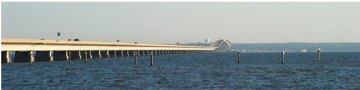
Figure 2-3. Mid-Bay Bridge, Choctawhatchee Bay, Florida (Worldbreak 2009).
