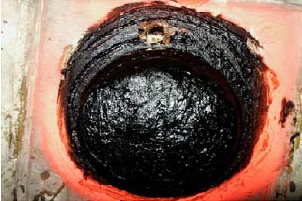
Figure K. Opened grout port.
