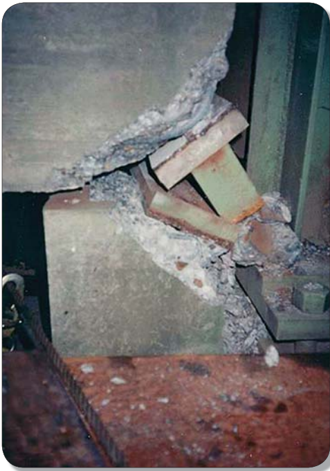
Figure 3.3: Failed Rocker Bearings (Yamhill River Bridge)
