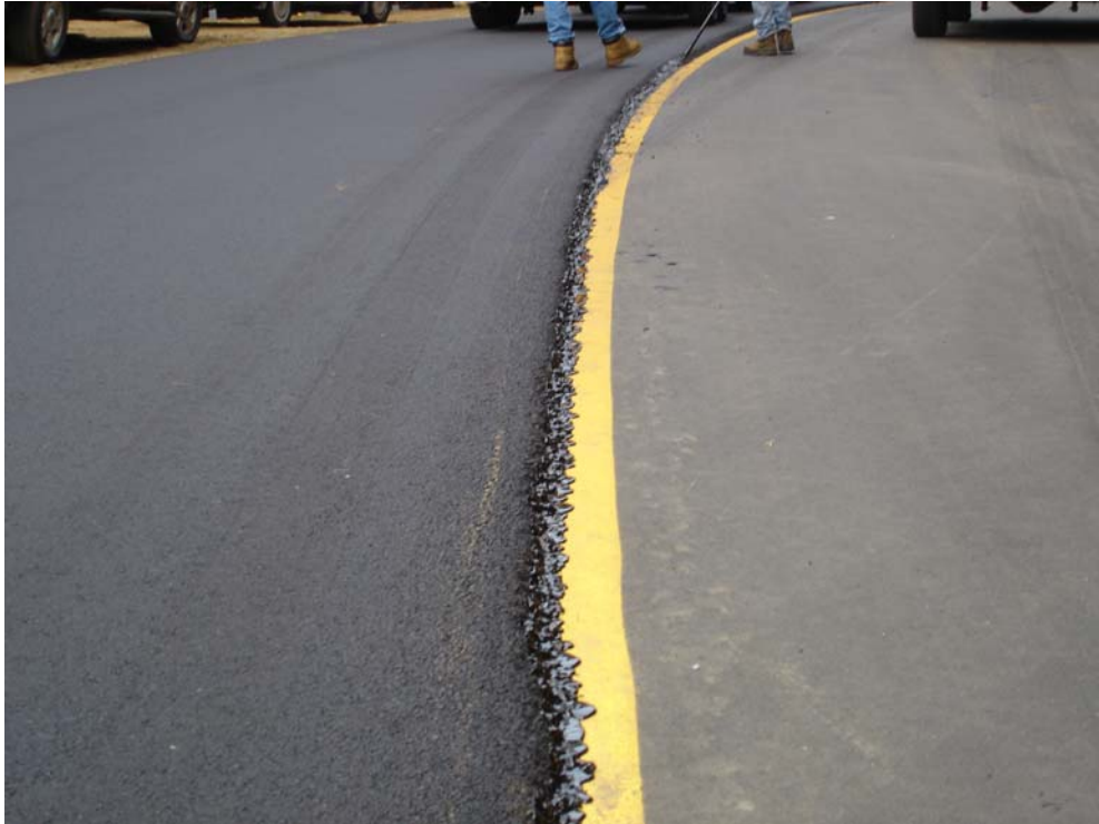
Figure 14 Rubberized Joint Sealant Applied to Cold Side of Joint
