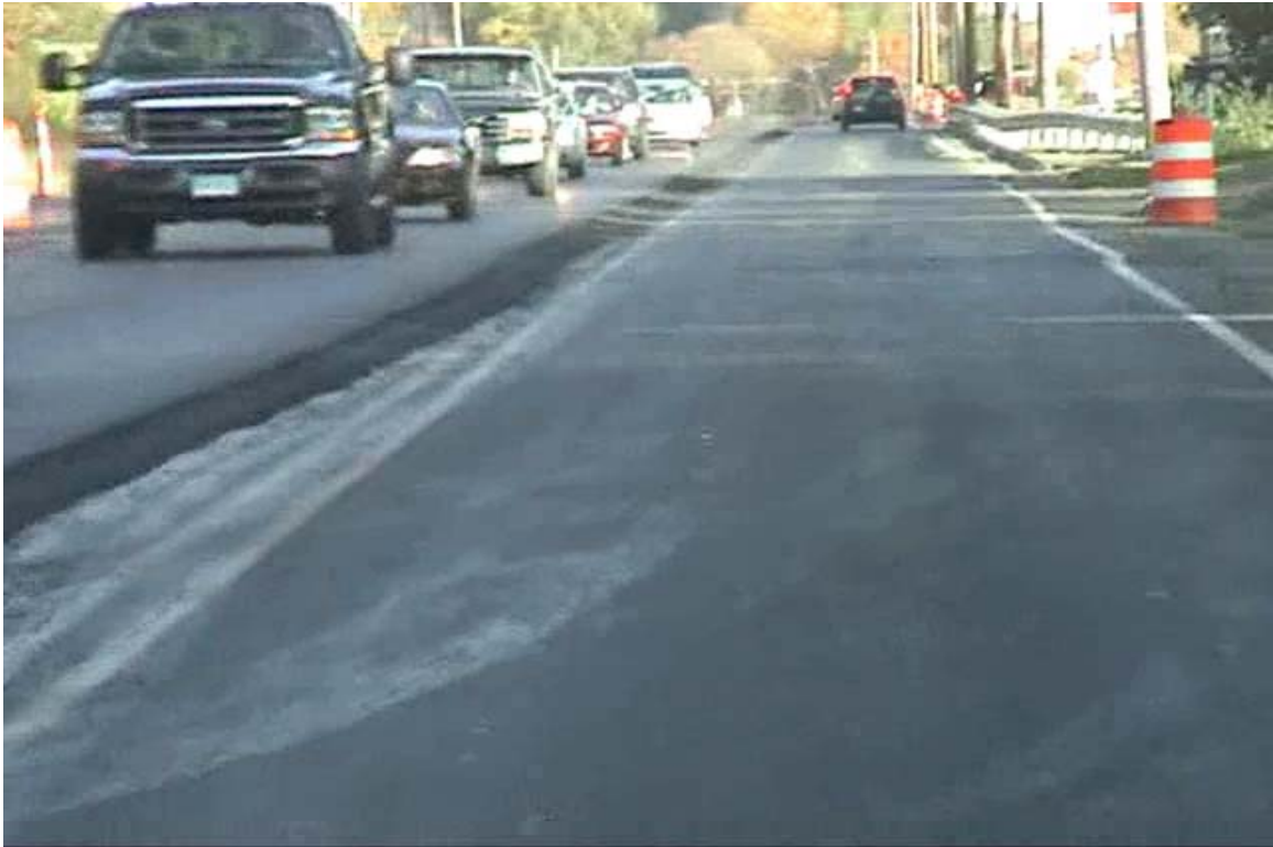
Figure 17 Traffic on Open Notched Wedge Joint
