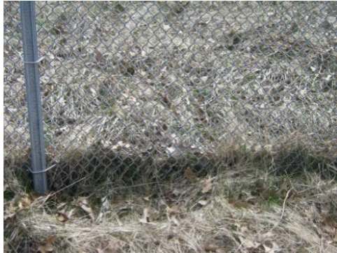
Figure 21 Cyclone Fencing Photo Credit: Stacy Cook
