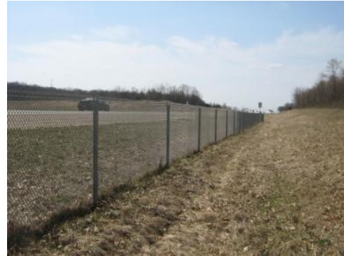
Figure 20 Cyclone Fencing Photo Credit: Stacy Cook
