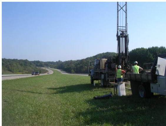
Figure 2: Subsurface Exploration Work at Site No. 9 (NOB-77)
