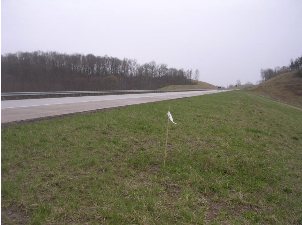
Figure 4.6: Highway Embankment Site No. 4 on USR 33 (Athens County)
