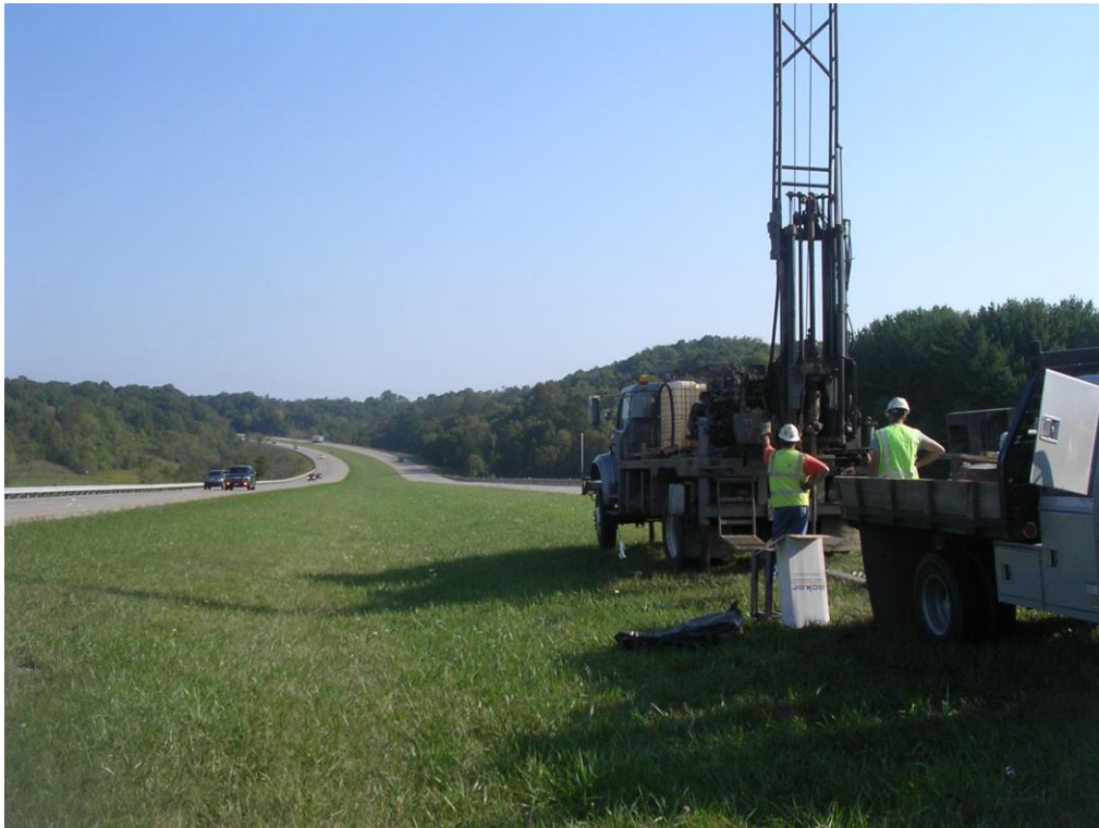
Figure 4.10: Highway Embankment Site No. 9 on I-77 (Noble County)
