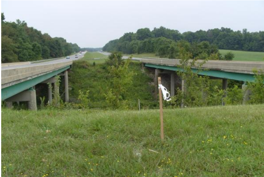
Figure 4.7: Highway Embankment Site No. 5 on I-71 (Morrow County)
