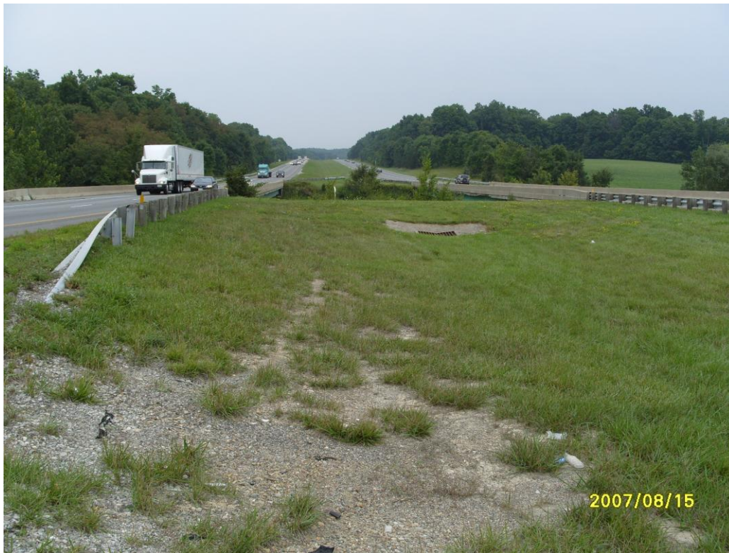
Figure 4.9: Highway Embankment Site No. 8 on I-70 (Muskingum County)
