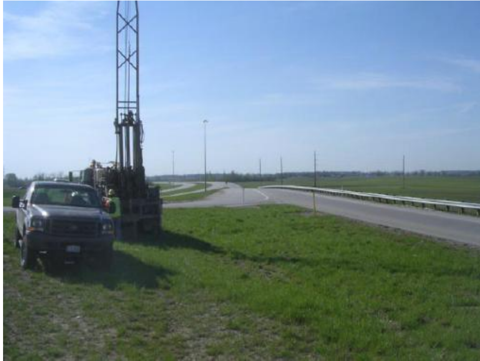
Figure 4.4: Highway Embankment Site No. 2 on USR 35 (Fayette County)
