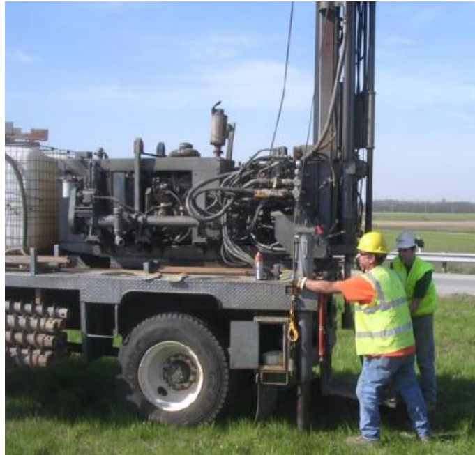
Figure 2.5: SPT Drill Rig Mounted on Back of Truck
