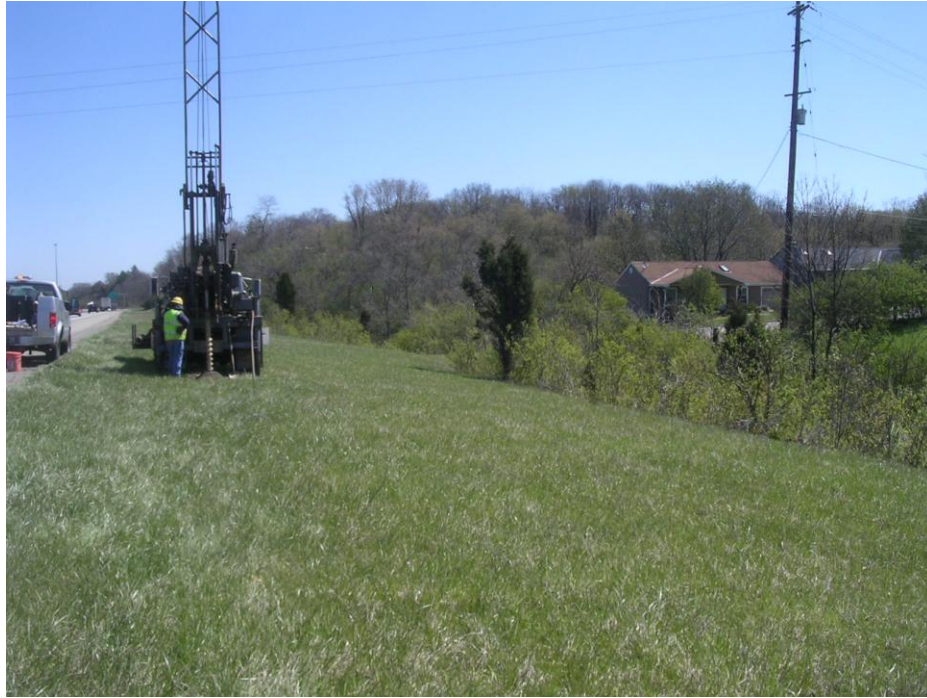
Figure 4.2: Highway Embankment Site No. 1 on I-275 (Hamilton County)
