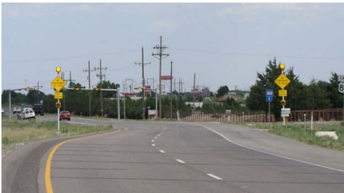
Figure 4. AWEGS Signs on a Two-Lane Approach.
