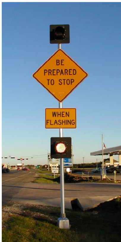
Figure 3. AWEGS Sign on a Single-Lane Approach.
