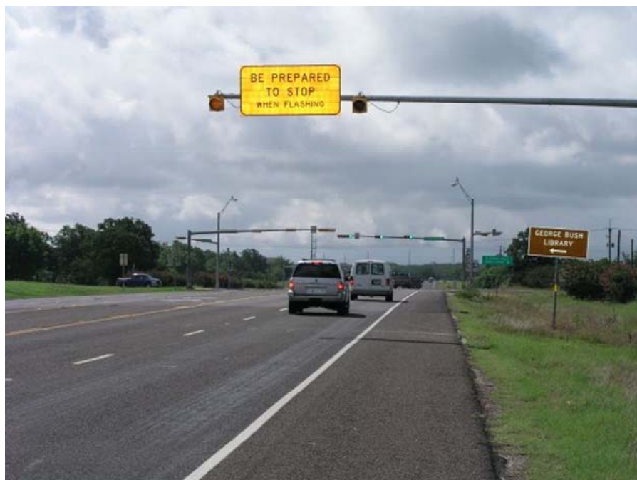
Figure 5. Overhead AWEGS Sign.
