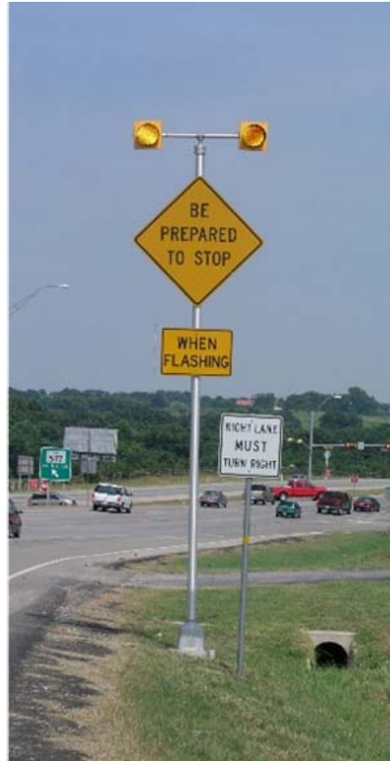
Figure 8. AWEGS Sign with the Beacons on Top.
