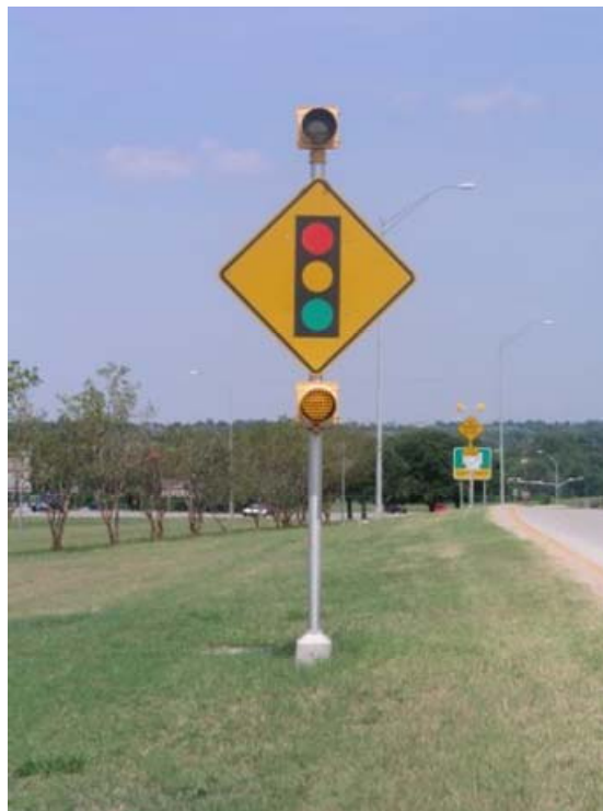
Figure 7. Signal Ahead Sign (W3-3) with Beacons.
