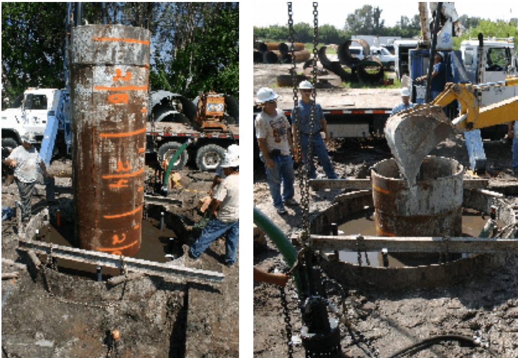
Figure 4-18. Placing and securing central casing.
