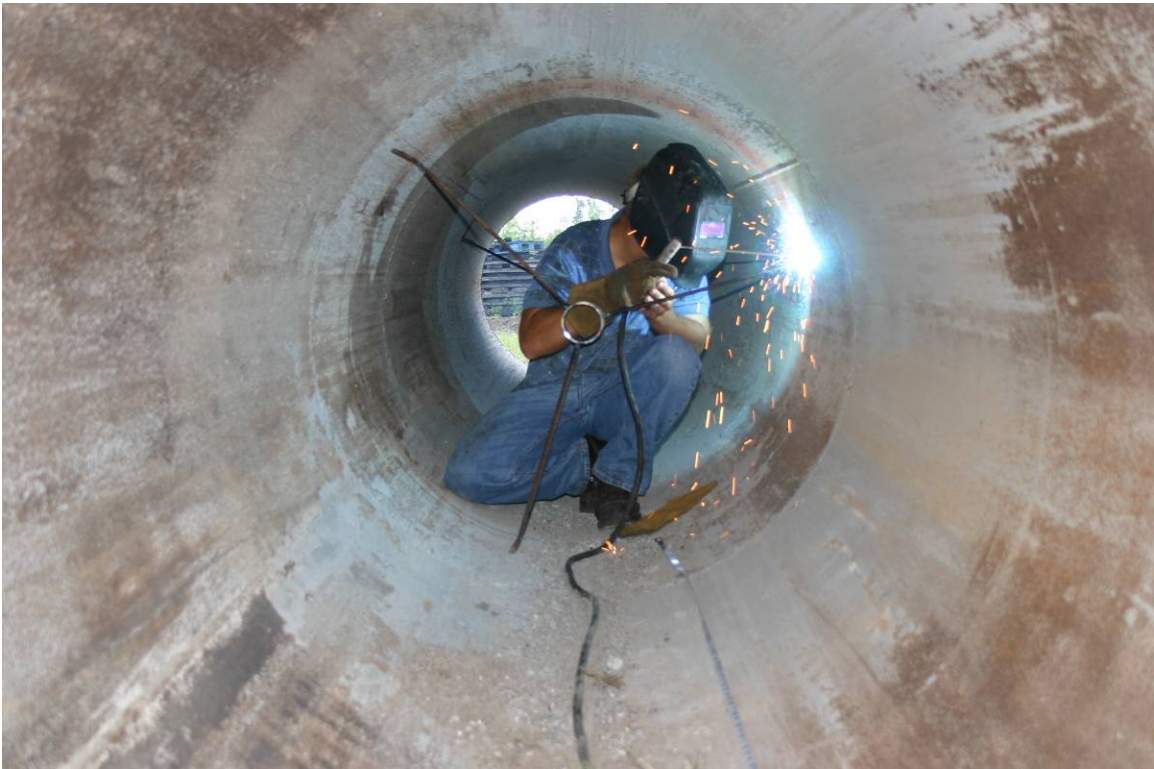
Figure 4-12. Voided shaft center casing access tube supports.
