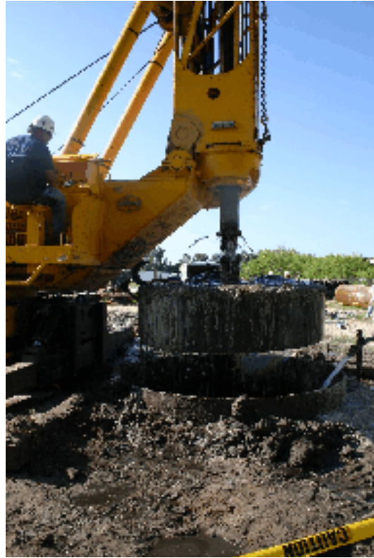
Figure 4-14. Drilling and clean-out of 9ft diameter excavation.
