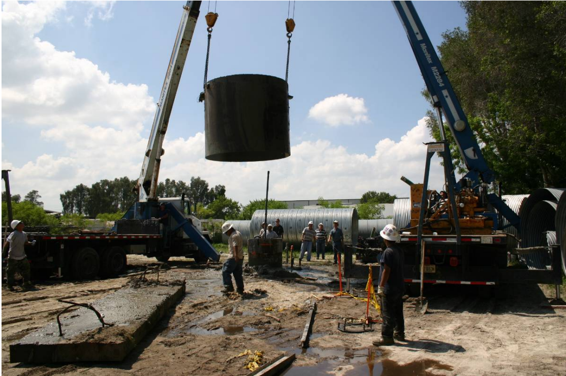
Figure 4-20. Temporary casing extraction.
