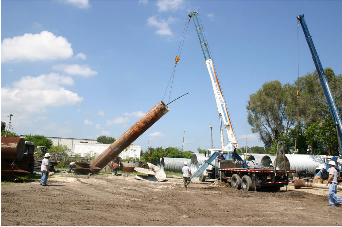
Figure 4-17. Lifting central casing.
