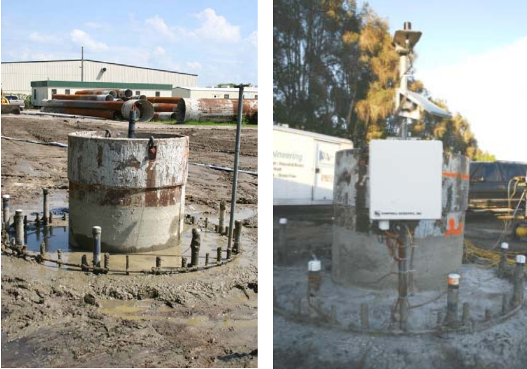
Figure 4-21. Finish shaft with data acquisition system in place.
