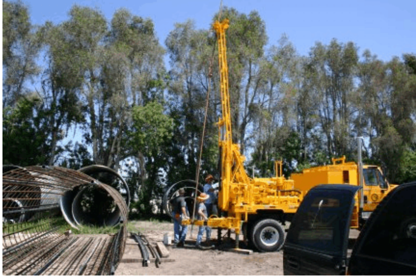
Figure 4-11. Installation of ground monitoring tubes by FDOT District I personnel.
