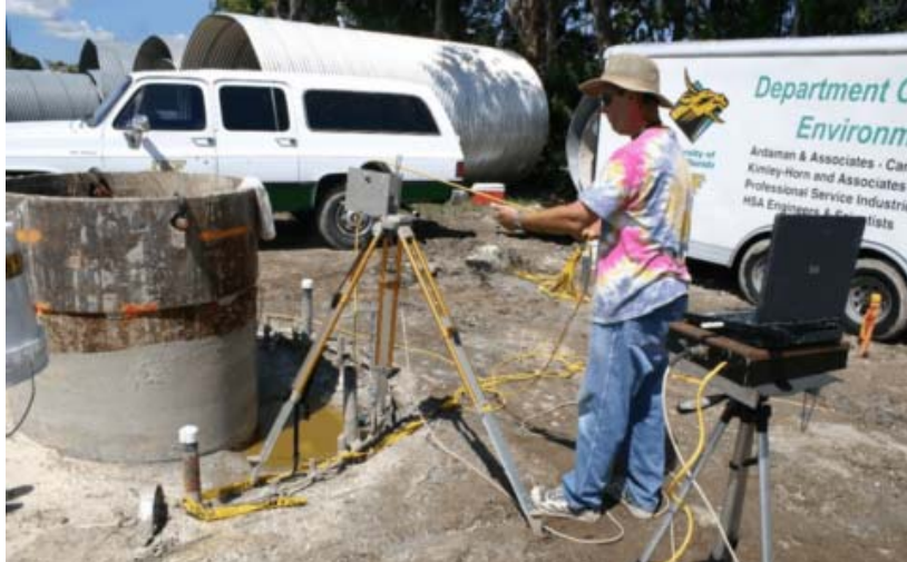
Figure 3-1. Thermal testing of voided shaft.
