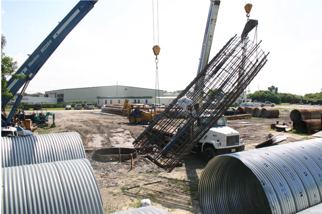
Figure 4-15. Lifting reinforcement cage.
