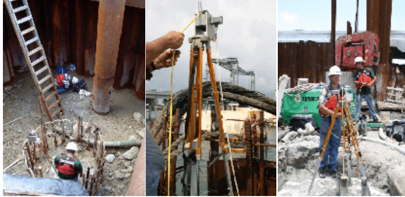
Figure 3-10. Thermal Integrity Testing of Shafts 6-2 (left), 8-2 (center), and 25-3 (right).
