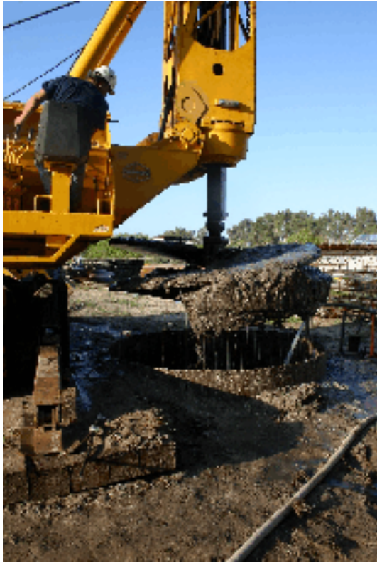
Figure 4-14. Drilling and clean-out of 9ft diameter excavation.
