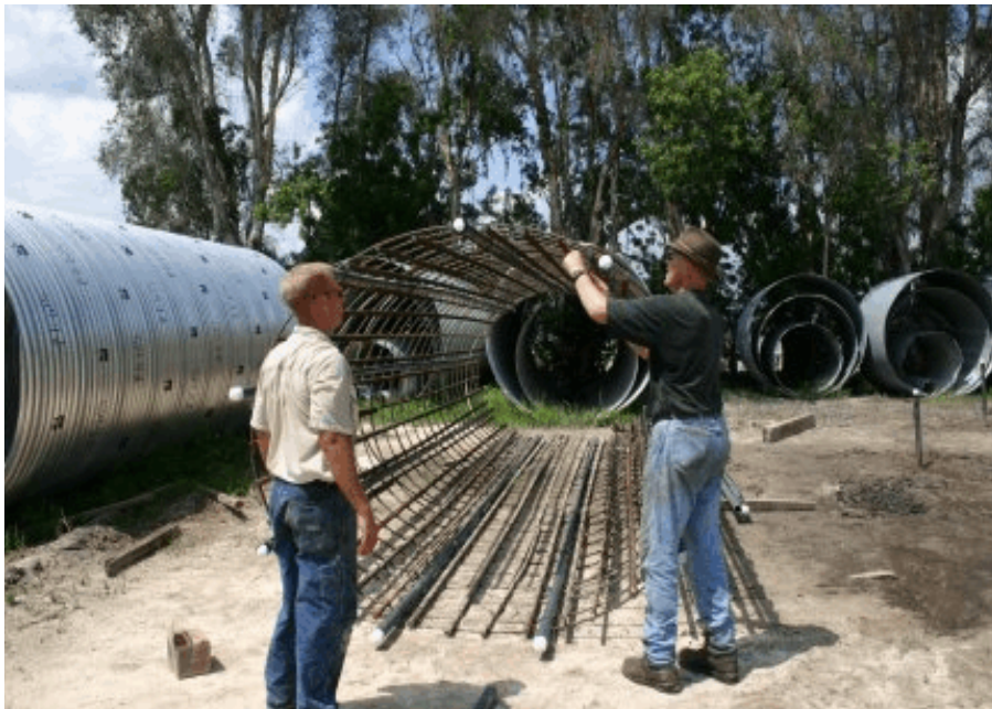
Figure 4-10. Reinforcement cage with monitoring tubes and thermocouples.
