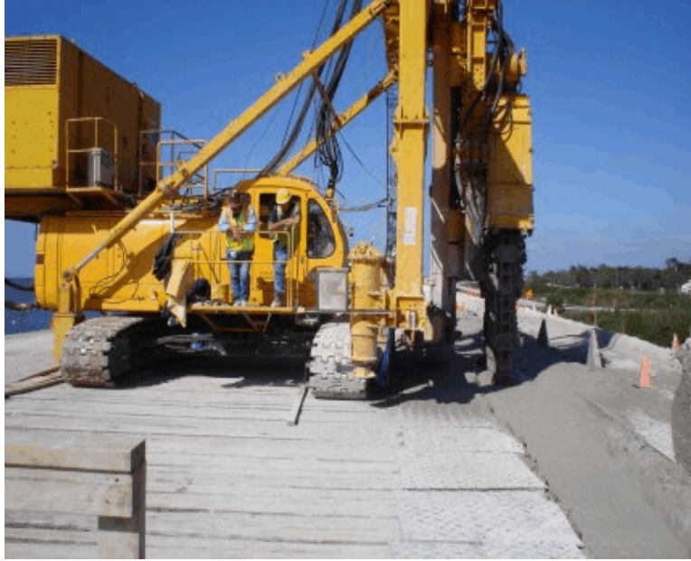
Figure 3-17. Lake Okeechobee dyke modifications using TRD.
