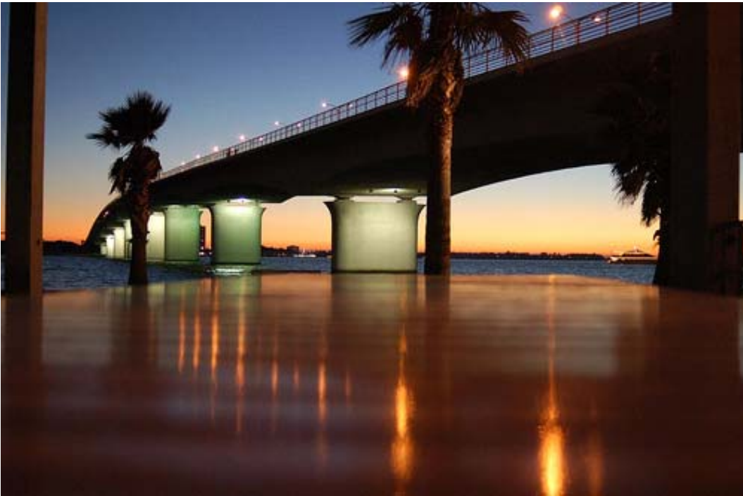
Figure 2-2. Ringling Causeway Bridge founded on 2- 9 ft diameter shafts at each pier.
