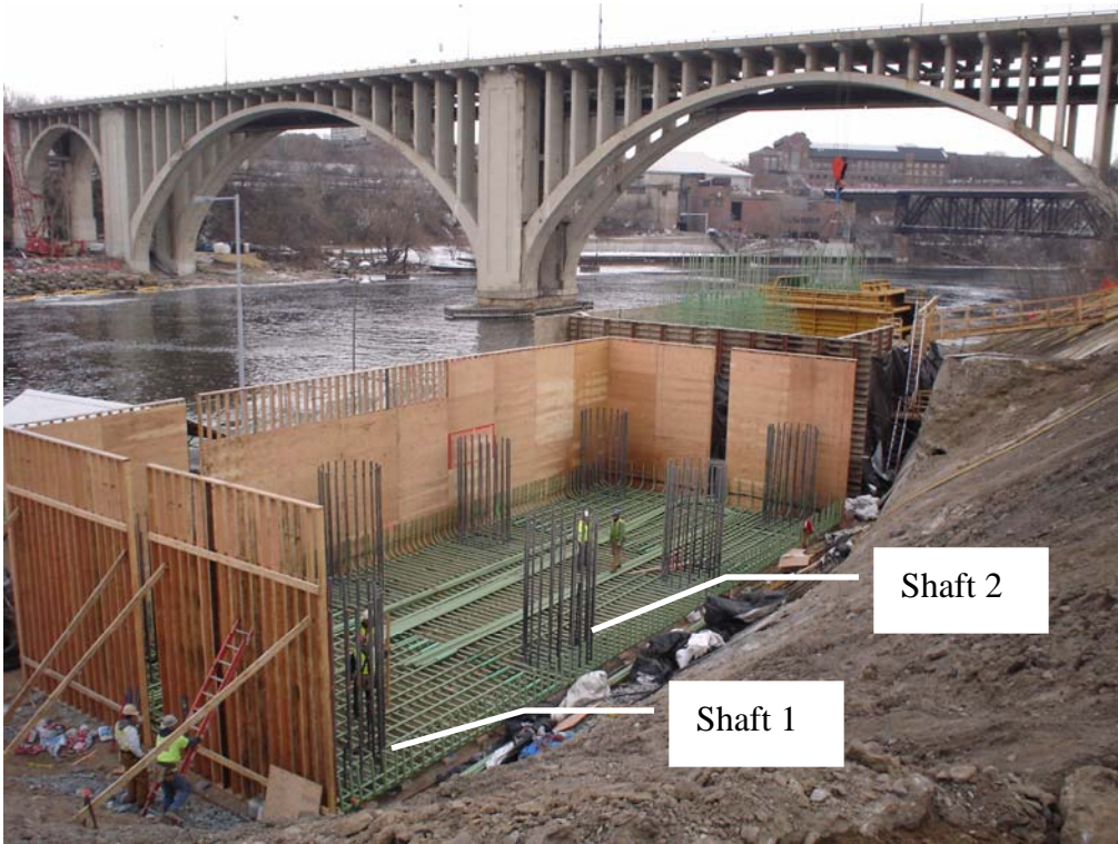
Figure 2-5. I-35W Bridge replacement southbound Pier 2.
