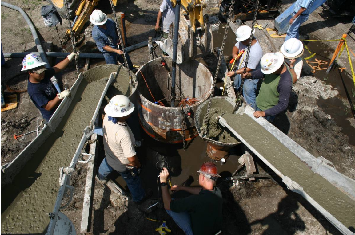
Figure 4-19. Concrete placement using two tremies.
