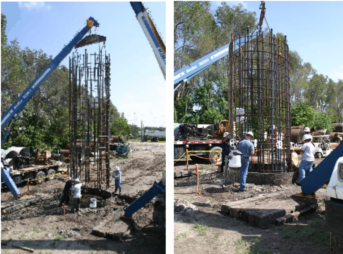
Figure 4-16. Placement of reinforcement cage with 12in diameter wheel spacers.
