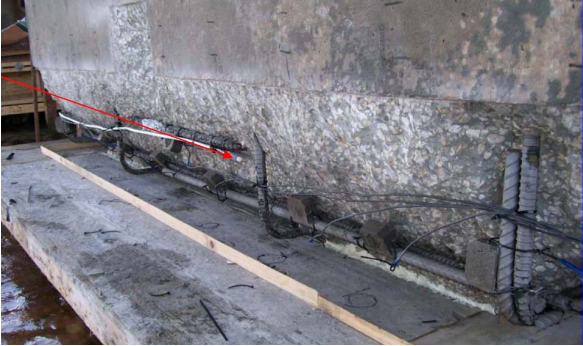
Figure 11 - Field Test Site 2, view of an instrumented Type W anode location before placing grout on anodes. Arrow shows position of an embedded reference electrode.
