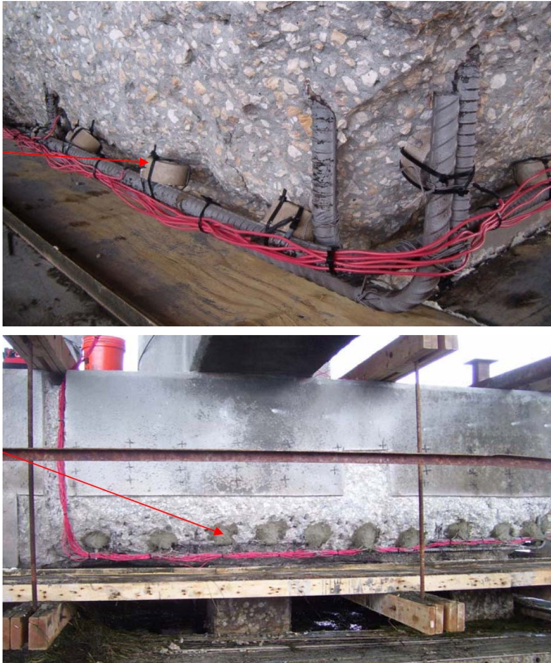
Figure 10 - Field Test Site 2, view of an instrumented Type C anode location before (top) and after placing grout on anodes (examples arrowed).
