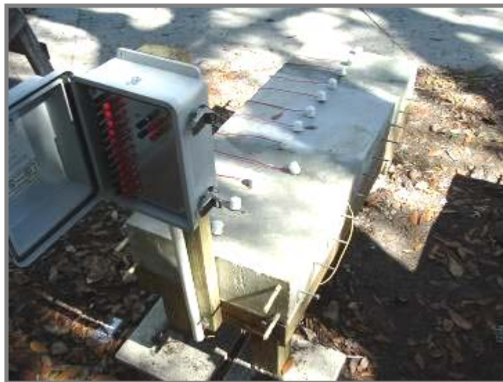
Figure 7 - Installed yard slab with connection box.
