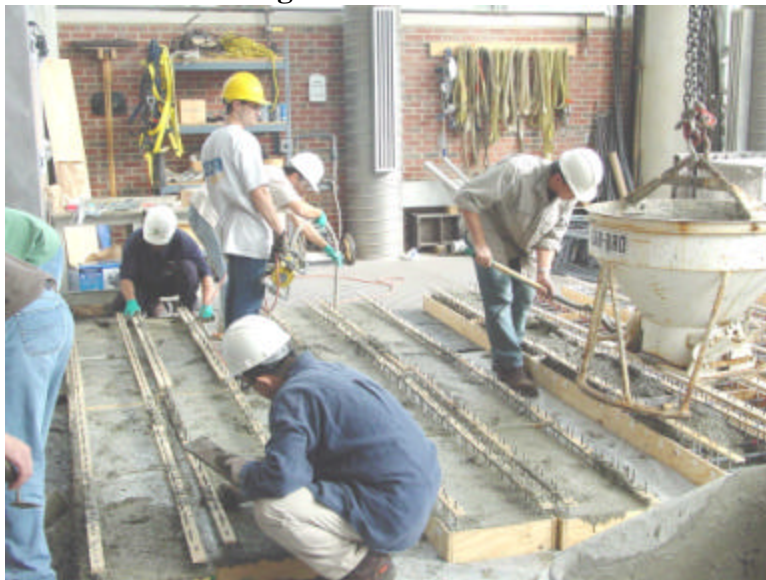
Figure 3.6 – Casting of the Slabs
