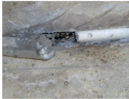
Filler material between Beams 6 & 7
