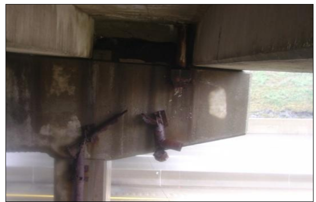
(b) damaged drain system resulting in water affecting superstructure (PennDOT).
