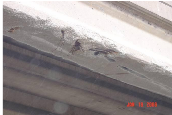
Span 3, Beam 8 – close up
