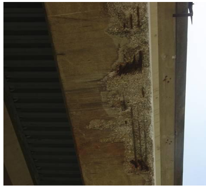
(b) close up view of (a) showing severed strands.
