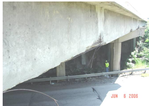
Beam 12 – Exposed strands near midspan, apparent impact damage
