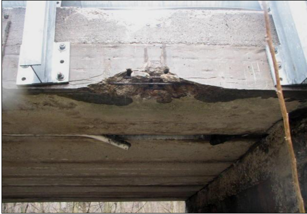
(a) spalling at original attachment and possible future damage at sight of new attachment
