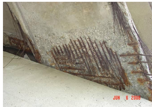
Beam 12 – Exposed strands near midspan, apparent impact damage
