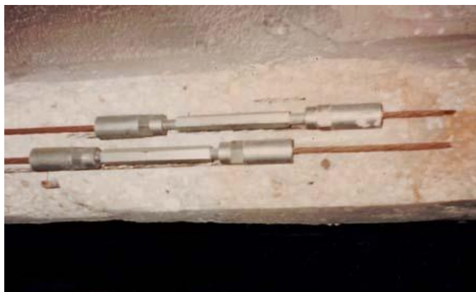
Figure 3.3 Commercially available 'turnbuckle' style strand splice (PCI.org)
