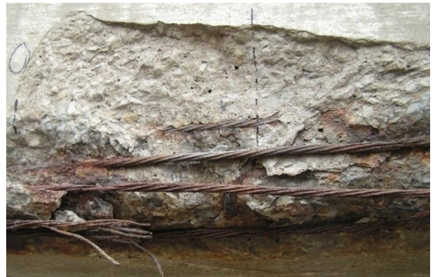
Figure 1.4 Exposed and ruptured strand due to vehicle impact (Lake View Drive Bridge; Harries 2006).
