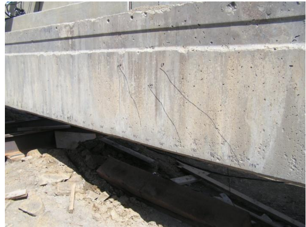
Figure 1.12 Representative shear distress (Lake View Drive EXTERIOR test girder; Harries 2006).
