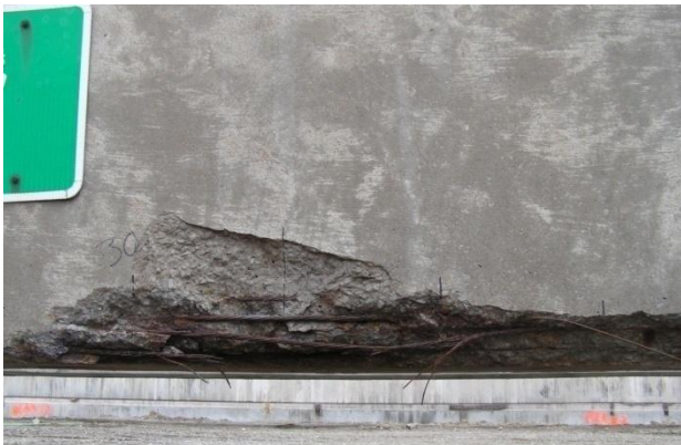
Figure 1.4 Exposed and ruptured strand due to vehicle impact (Lake View Drive Bridge; Harries 2006).
