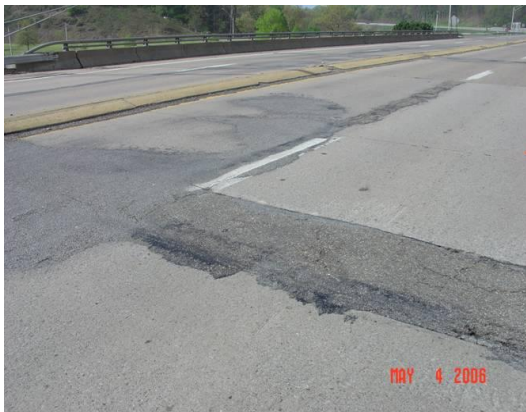
Far approach relief joint and approach slab
