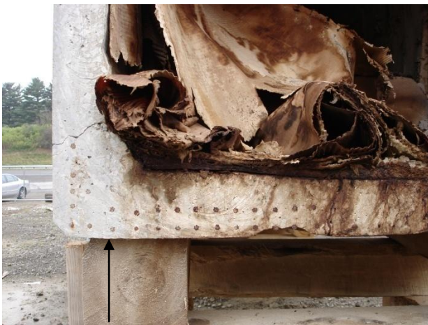
\frac{3}{4} " center of strand to soffit
