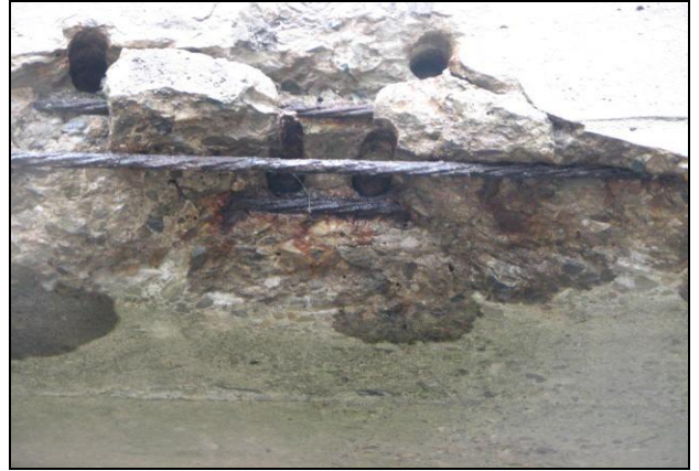
(b) unpatched holes at sight of original attachment result in exposed strands.
