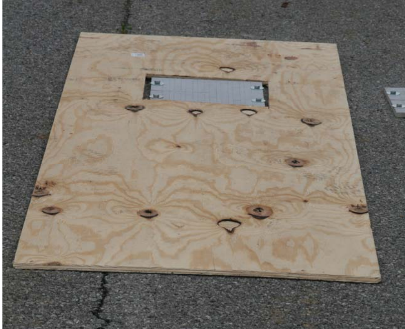
Figure 5. Plywood Covering Sample Test Plates.
