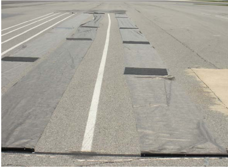
Figure 13. Layout of Experimental Pavement Markings with Landscaping Paper.
