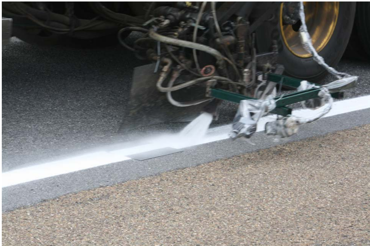
Figure 3. Photograph of Pavement Marking Application Process. (Photograph taken during calibration procedure)
