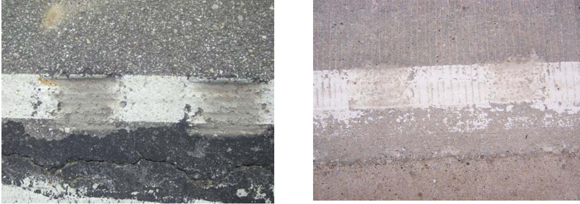
Figure 5-4. Swept stripe areas on asphalt and PCC pavements
