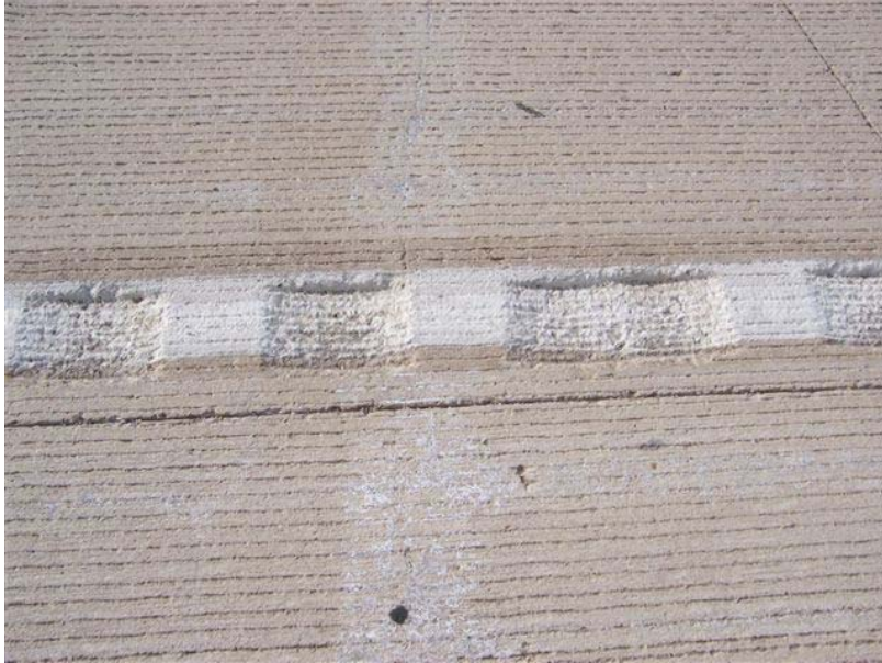
Figure 5-16. Similar wear for rumble stripe and flat section on E-16 (taken spring 2009)
