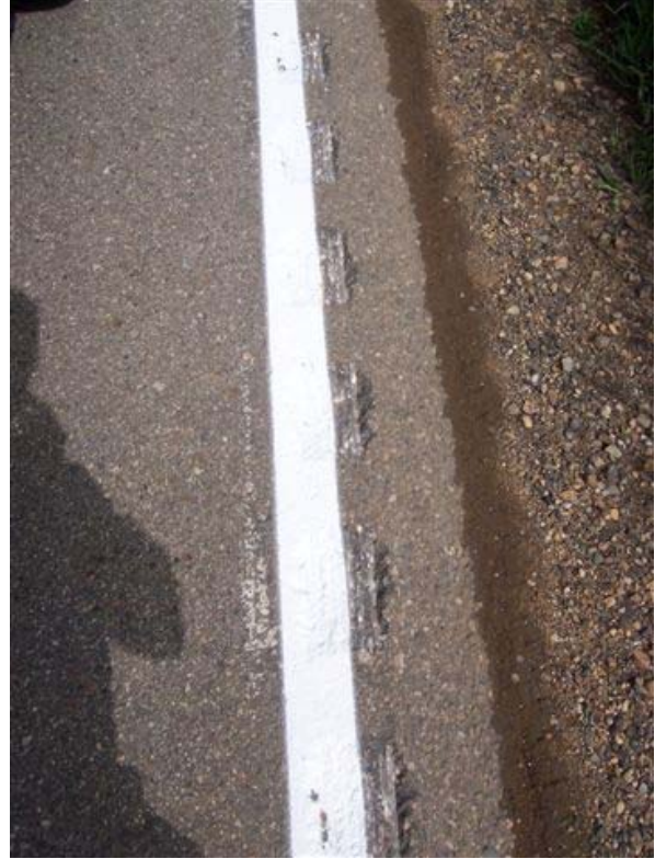
Figure 3-14. Photos showing difficulty in maintaining painted edge line alignment within rumble stripe installation
