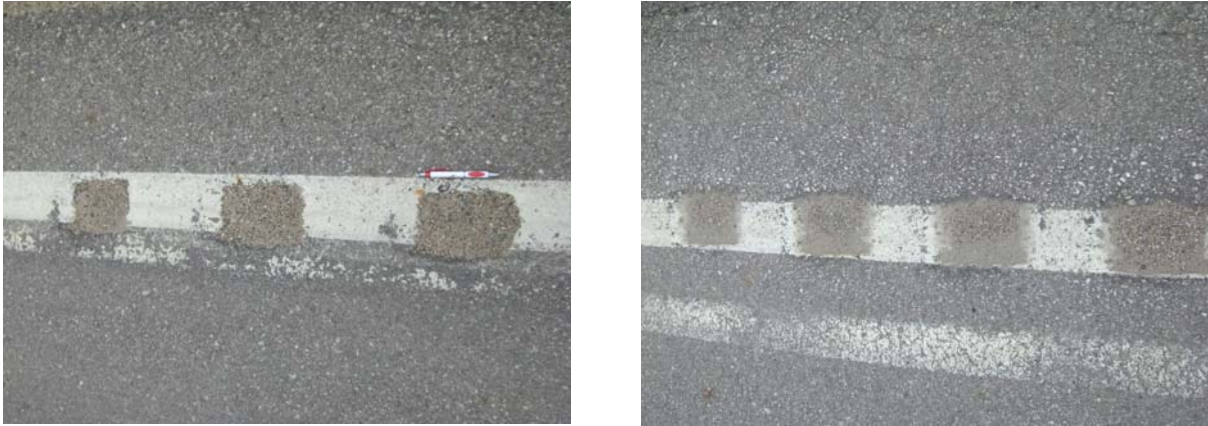
Figure 5-2. Rumble stripes filled with sand
