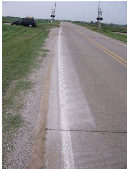
Figure 4-6. Rumble stripe installation on P-53
