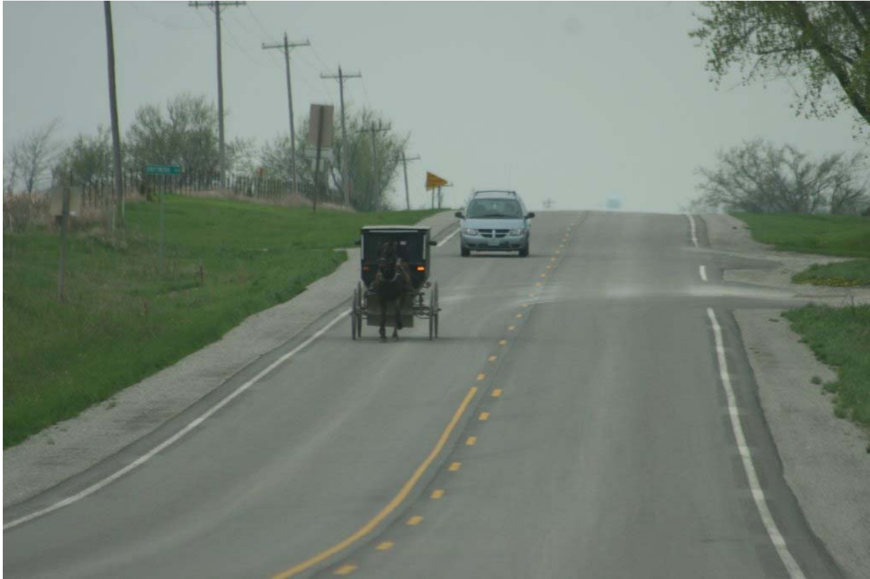
Figure 5-21. Edge line rumble strips in place along Iowa 2 (image courtesy of Neal Hawkins, CTRE)
