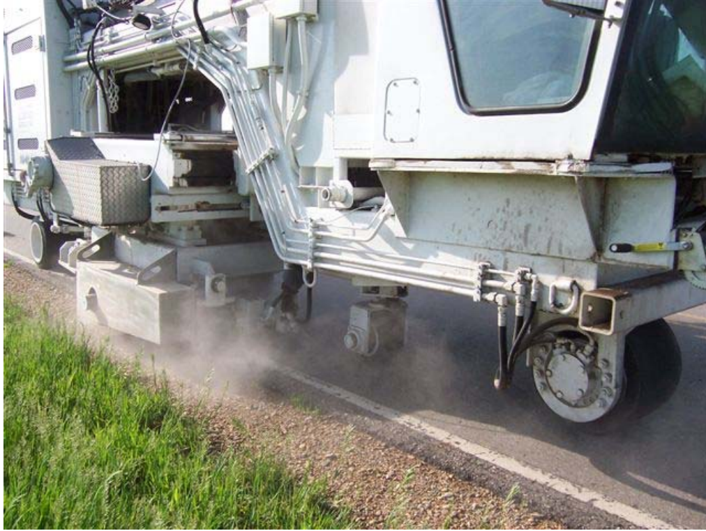
Figure 3-5. Close-up of the milling process
