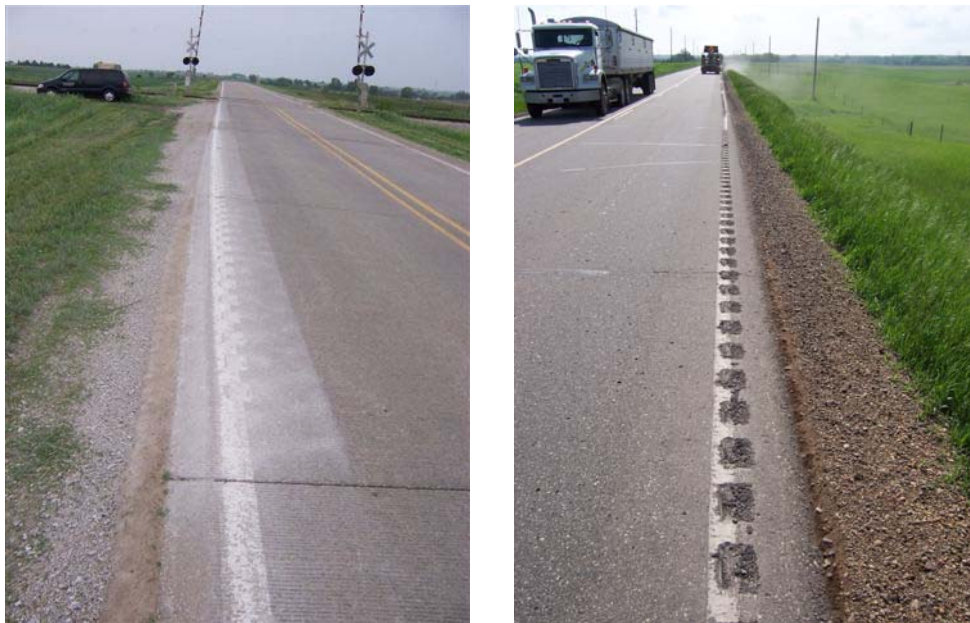
Figure 3-9. Examples of milling work
