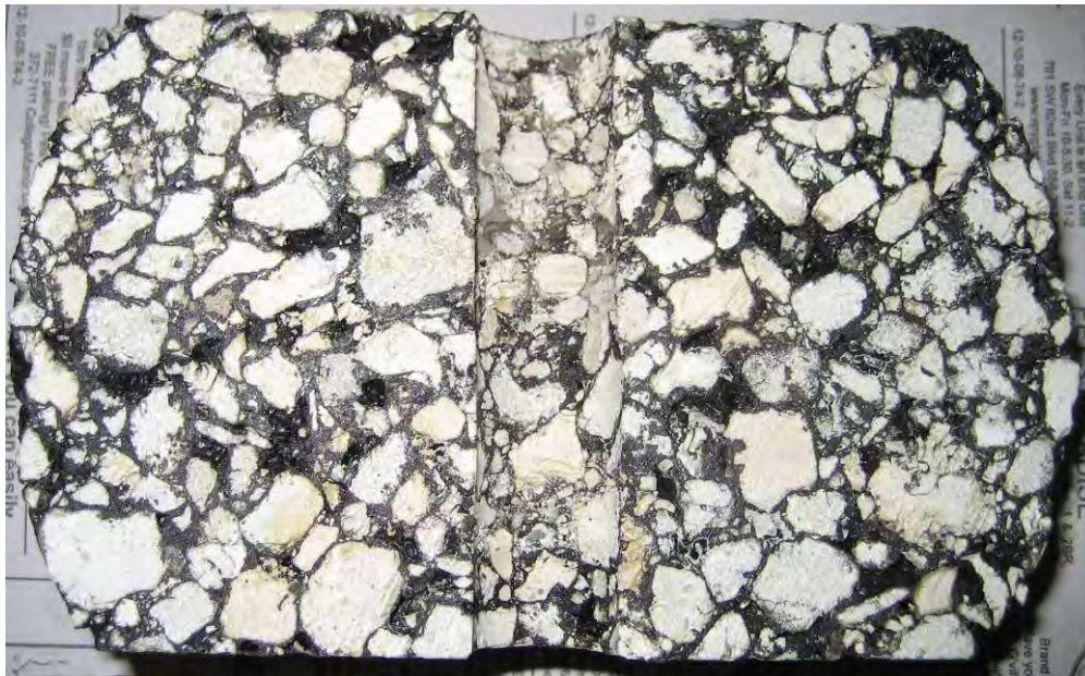
Figure 5-33 Compacted Open-Graded Mixture Surface After Slicing
