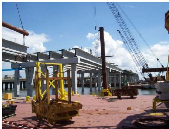
I-10 Twin Span Bridge Construction
