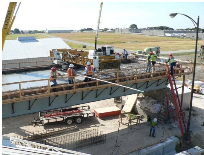
Figure 3.8: Photograph of instrumented bridge prior to deck placement
