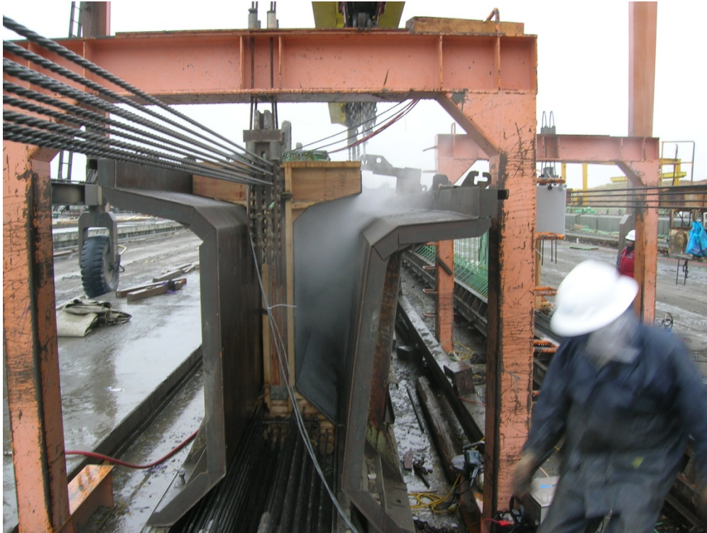
Figure 3-3 Girders were cured in steel forms with no external steam
