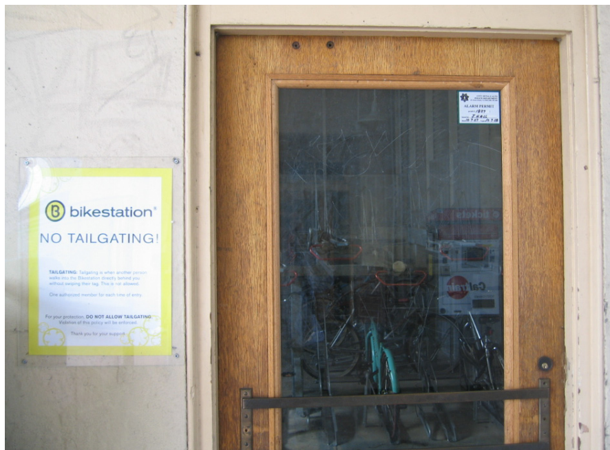
Figure 15. Bike storage room at Stanford University transit center.
