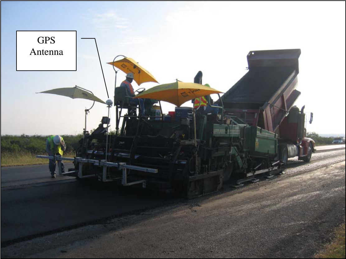
Figure 3. Pave-IR with GPS on Paver at US 90 Project.
