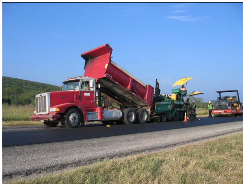
Figure 2. Paving CAM on US 90.
